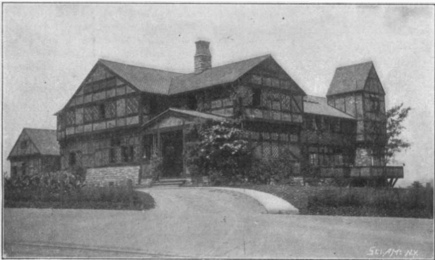
VIEW OF THE WORKS.
