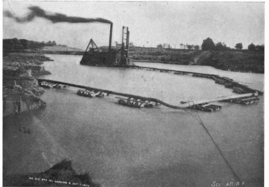
Large Hydraulic Dredge at Work, Showing Floating Discharge Pipe.
