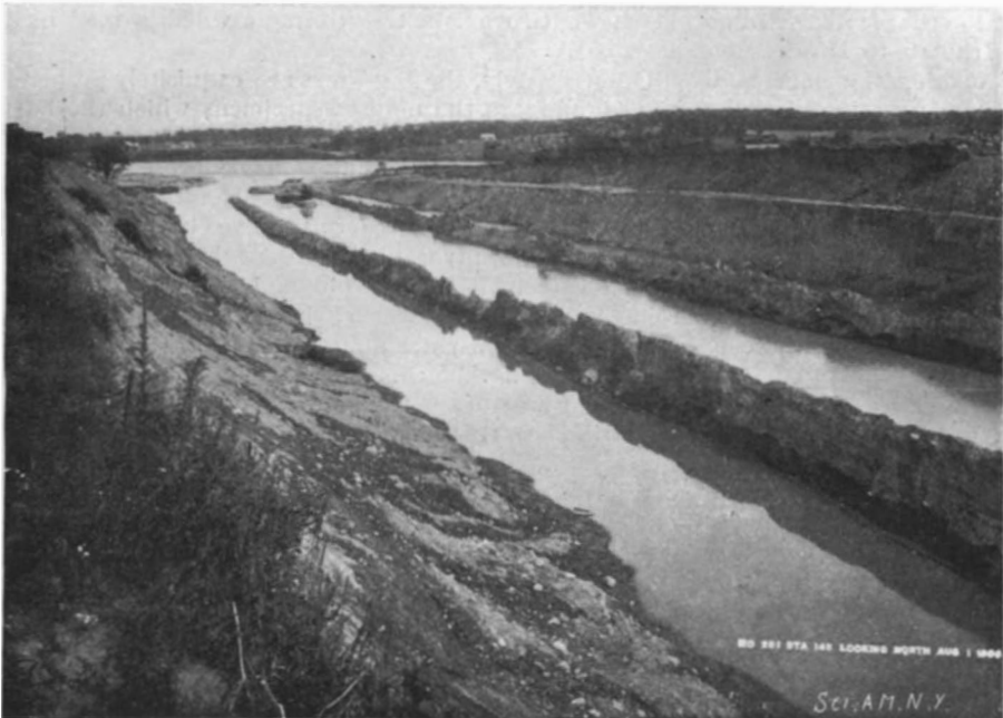
Partially Completed Canal (August 1) at Entrance from St. Lawrence River.
