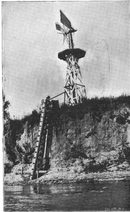
WATER ELEVATOR ON BLUE RIVER, NEBRASKA.
