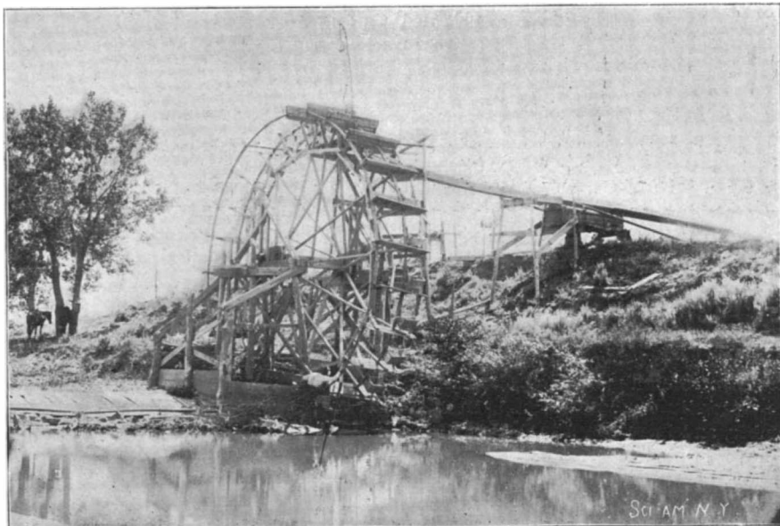
30-FOOT CURRENT WHEEL ON BRANCH OF HOT CREEK, NEBRASKA.
