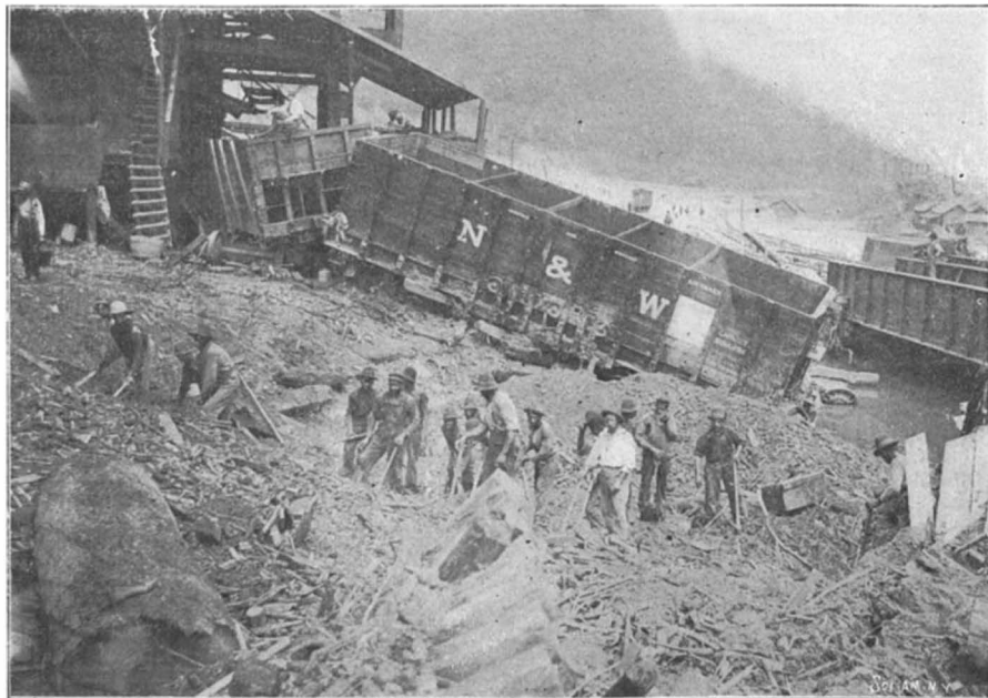
Freight Train Destroyed by the Flood.
