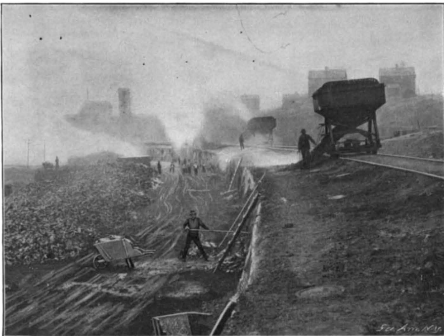
Charging, Drawing, and Loading Coke.
