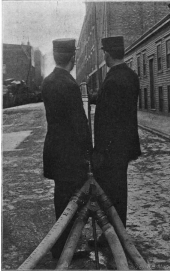
FOUR-WAY CONNECTION ATTACHED TO NOZZLE.
