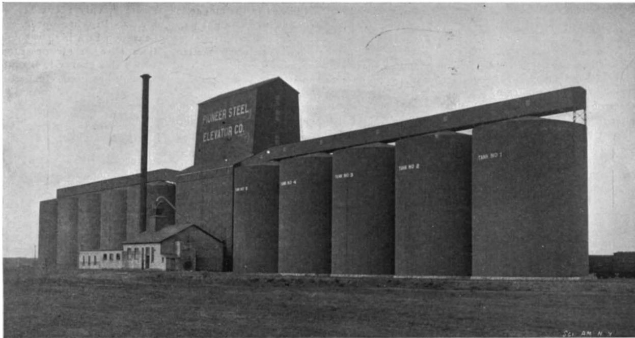
FIREPROOF STEEL TANK ELEVATOR OF 1,200,000 BUSHELS CAPACITY.
