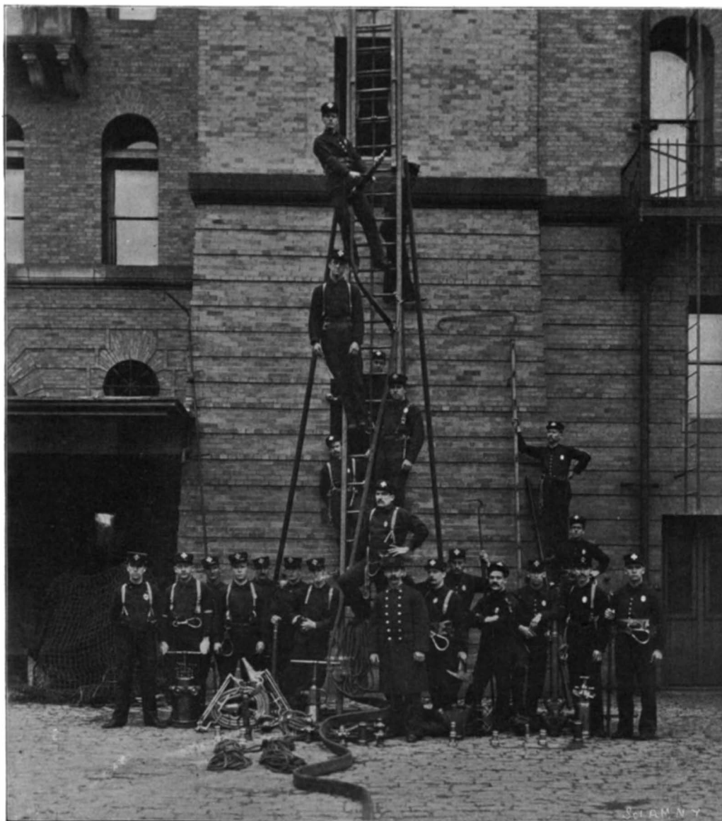
BOSTON FIRE-DRILL SCHOOL—FIREMEN READY TO PERFORM EVOLUTIONS.
