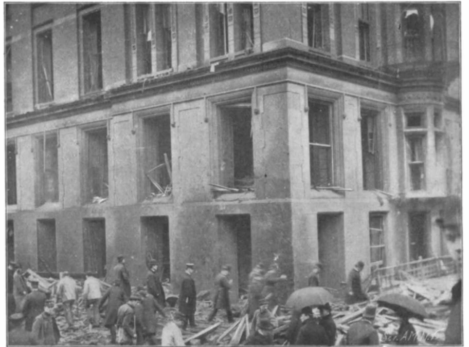
Northeast Corner of Murray Hill Hotel, Which Felt Full Blast of Explosion.
