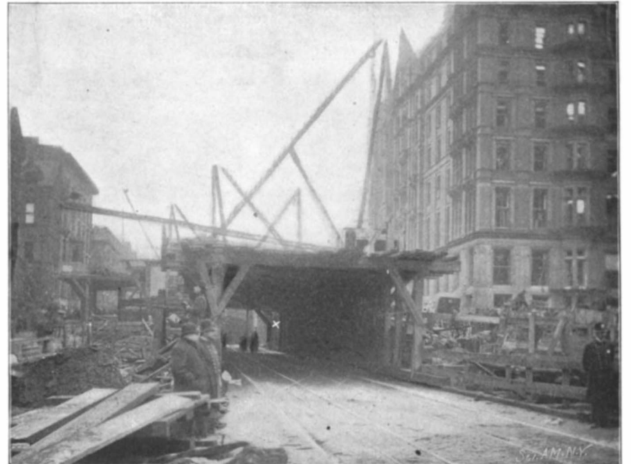
Looking South Toward Park Avenue with Subway Excavation at the Right of Tunnel.
