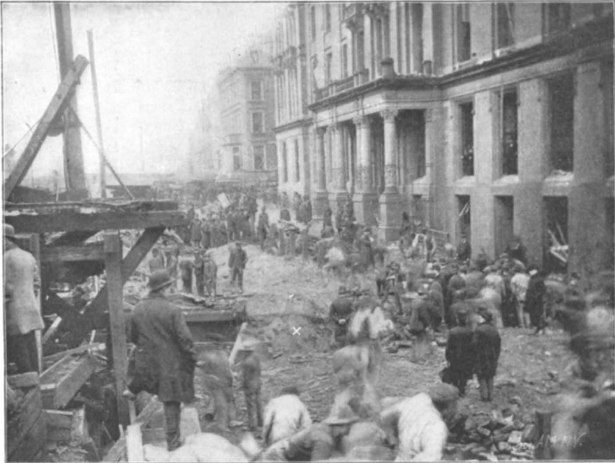
Looking South on Park Avenue. Cross Indicates Location of Dynamite.
