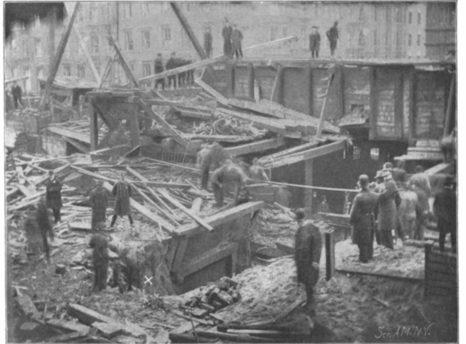
Exact Locality of Explosion Showing Openings into the Subway and Park Avenue Tunnel.
