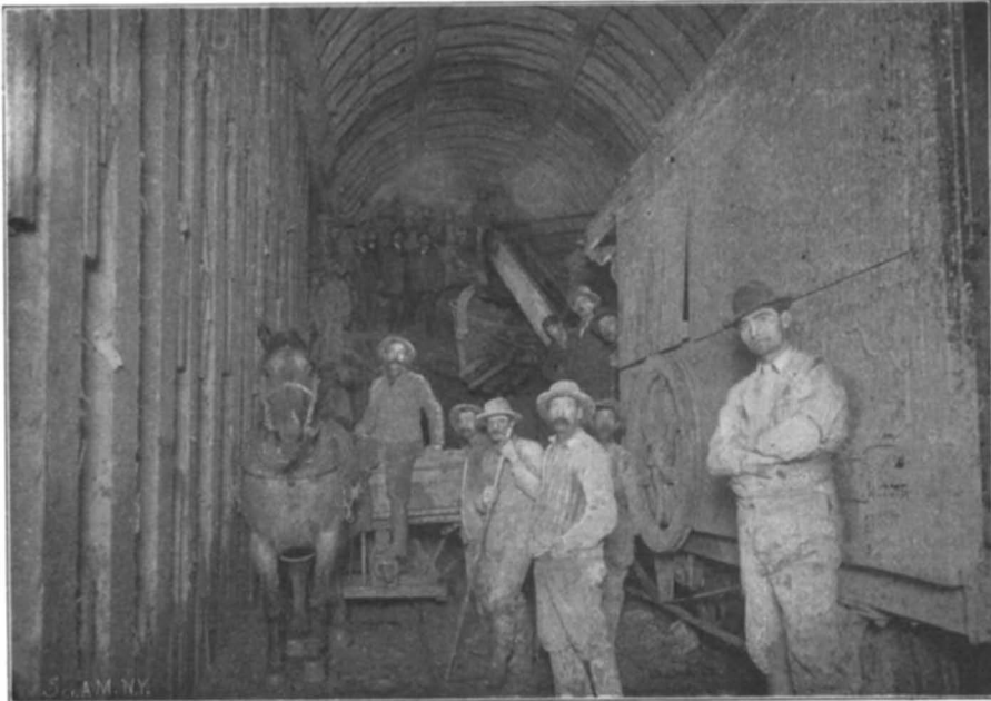
West End Shovel Taking up Muck from Bench.
