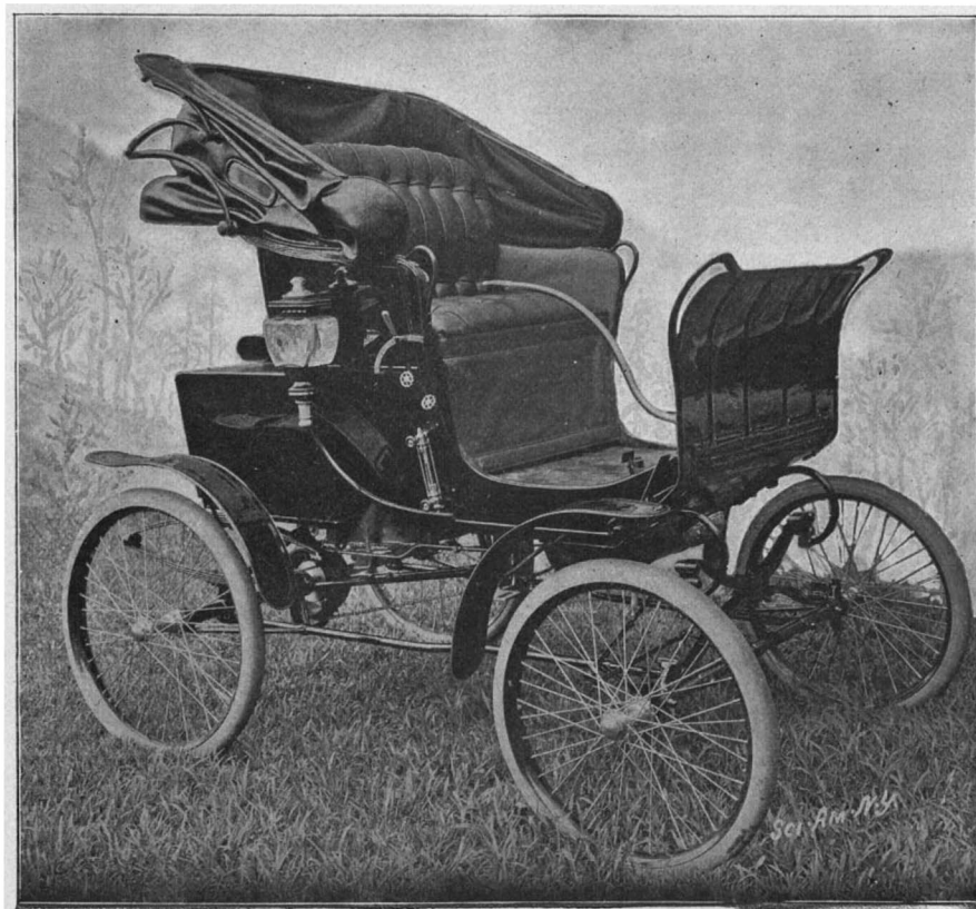
THE GROUT STEAM STANHOPE.
