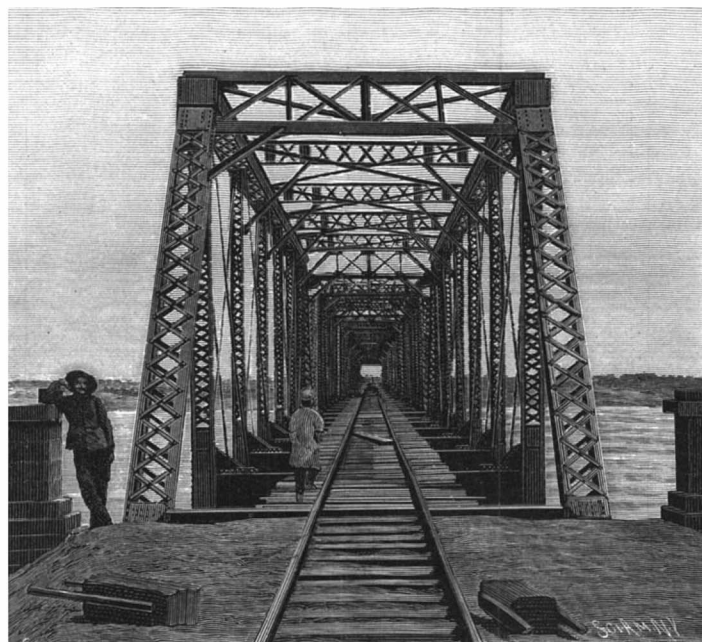
PORTAL VIEW OF THE COMPLETED BRIDGE.
