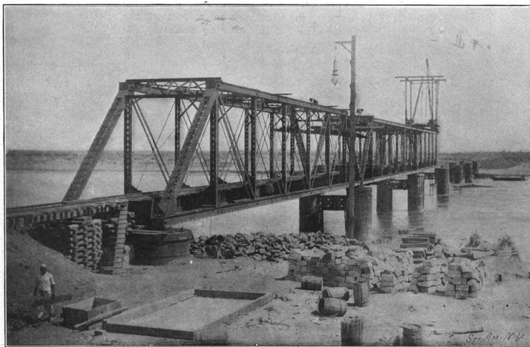
Seven 147-foot spans; total weight of superstructure, 620 tons. Order received January 20; structure shipped March 7; erection completed August 19.
