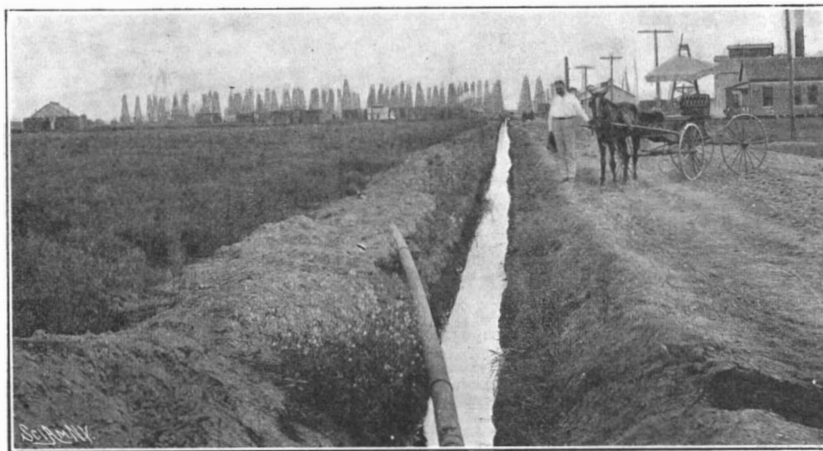
A Typical Pipe Line, and an Open Ditch for Conveying Oil to the Earthen Reservoir
