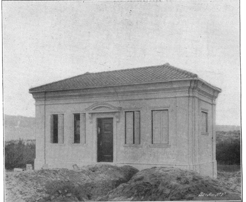
Landing Station of Pacific Cable, on Ocean Beach, San Francisco.
