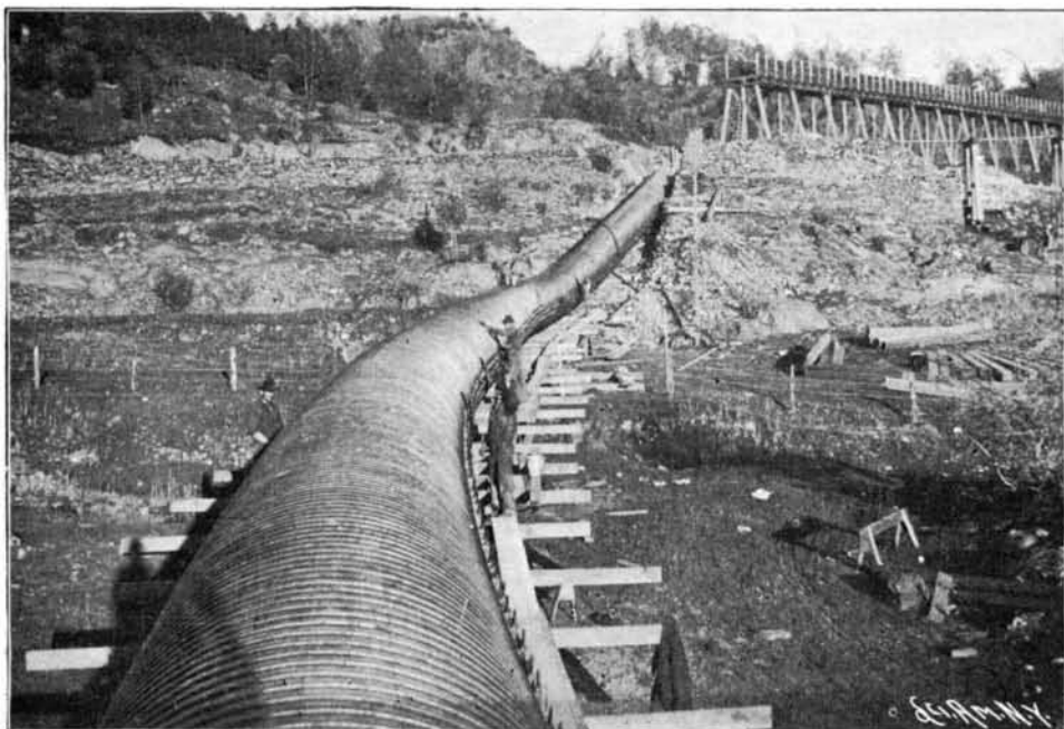
Redwood Stave Pipe that has Supplanted an Irrigation Flume.
