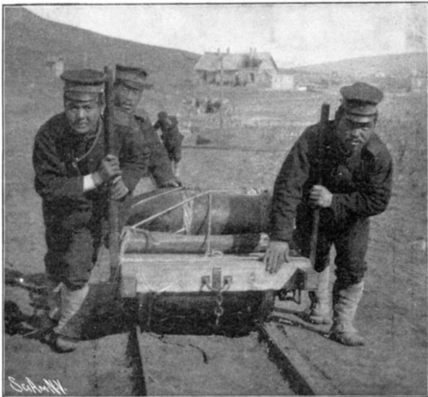
The mortars, their mounts, and the materials for the concrete emplacements, were all brought to the site of the batteries over a narrow-gage road, which was under fire for two months.
