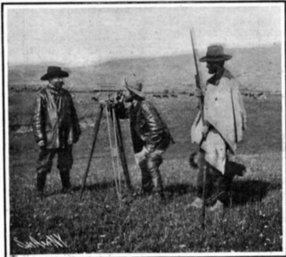
Leveling the Tulcan Base.
