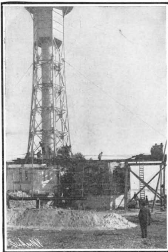
Lighthouse During Removal.
