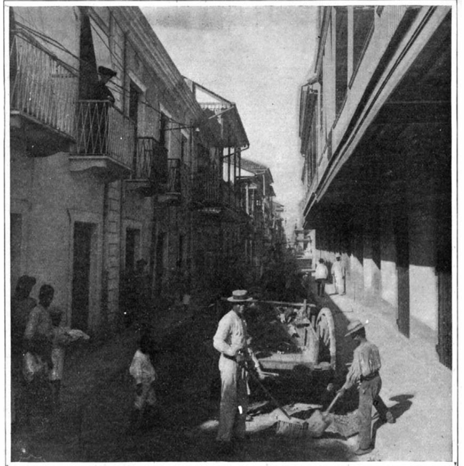
Street Cleaning Department at Work on One of the Streets of Panama. This Street Has Been Graded and Covered with Top Dressing of Gravel.
