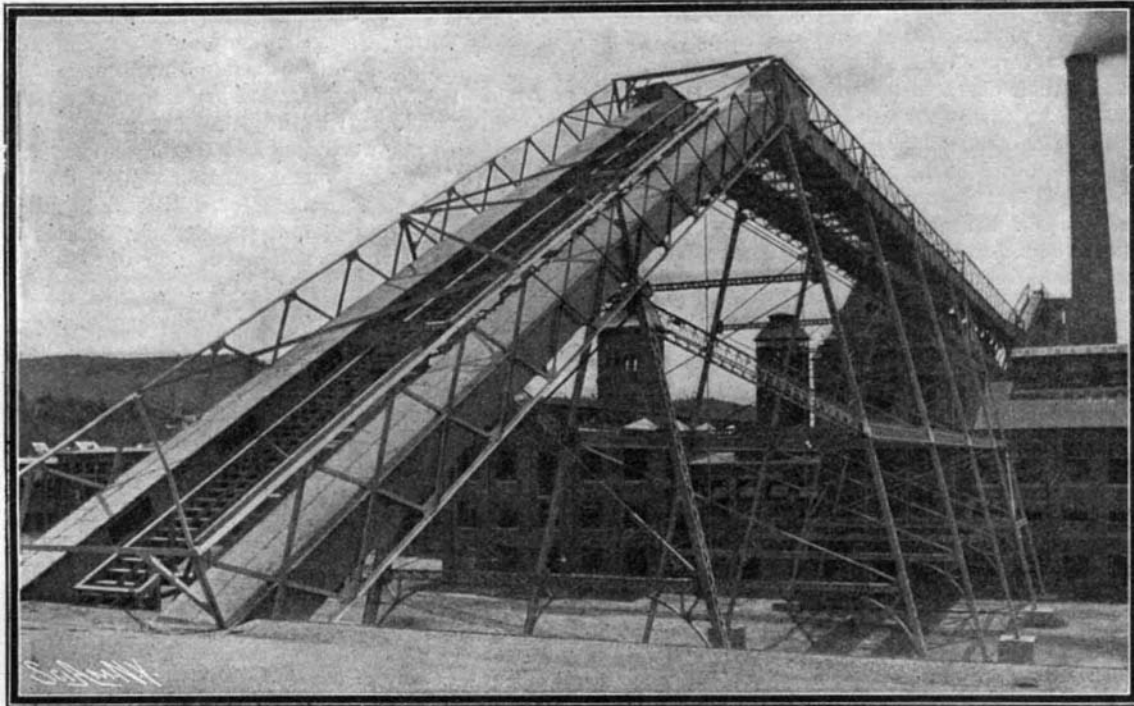
A 1,500-Foot Conveyer Used in Connection with a Pulp Plant.
