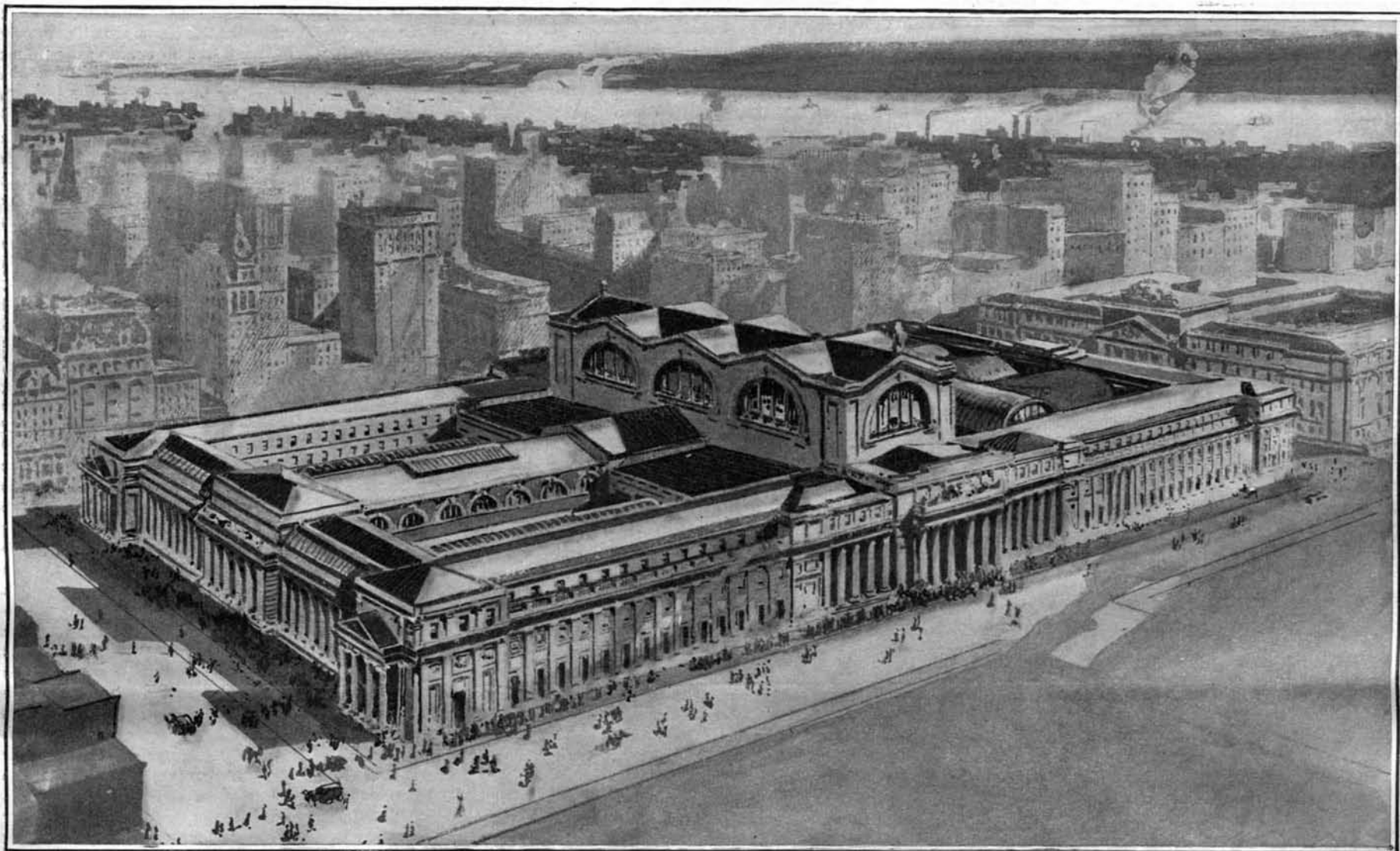
Bird's Eye View of Station From the Northeast as It Will Appear When Completed.
