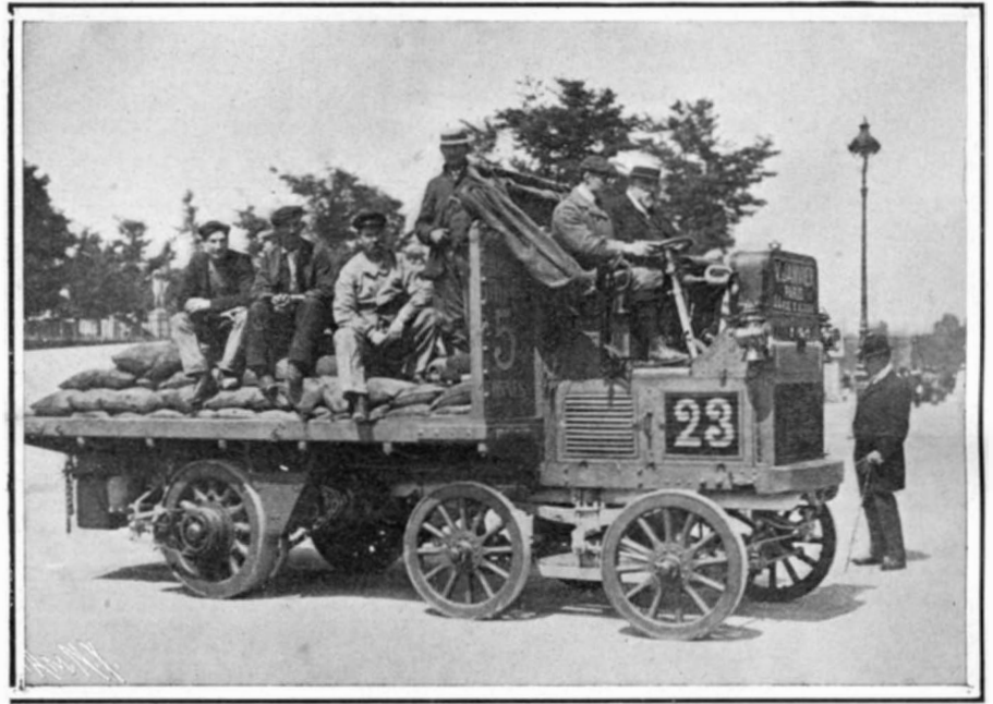
The 3-Cylinder, 24-Horse-Power Janvier Truck, Fitted with Novel Steering Bogie.
