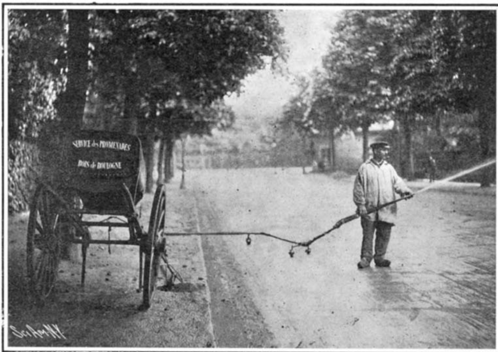
Sprinkling with Oil by Means of a Portable Mixer.
