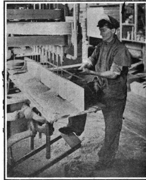
Fig. 8.—One of Several 11-Gang Drills, Boring Air Ducts in Edge of Well-Board.
