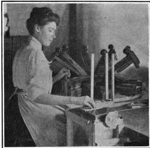
Fig. 6.—Press for Glueing Sheepskin Diaphragms on the Power Pneumatics.
