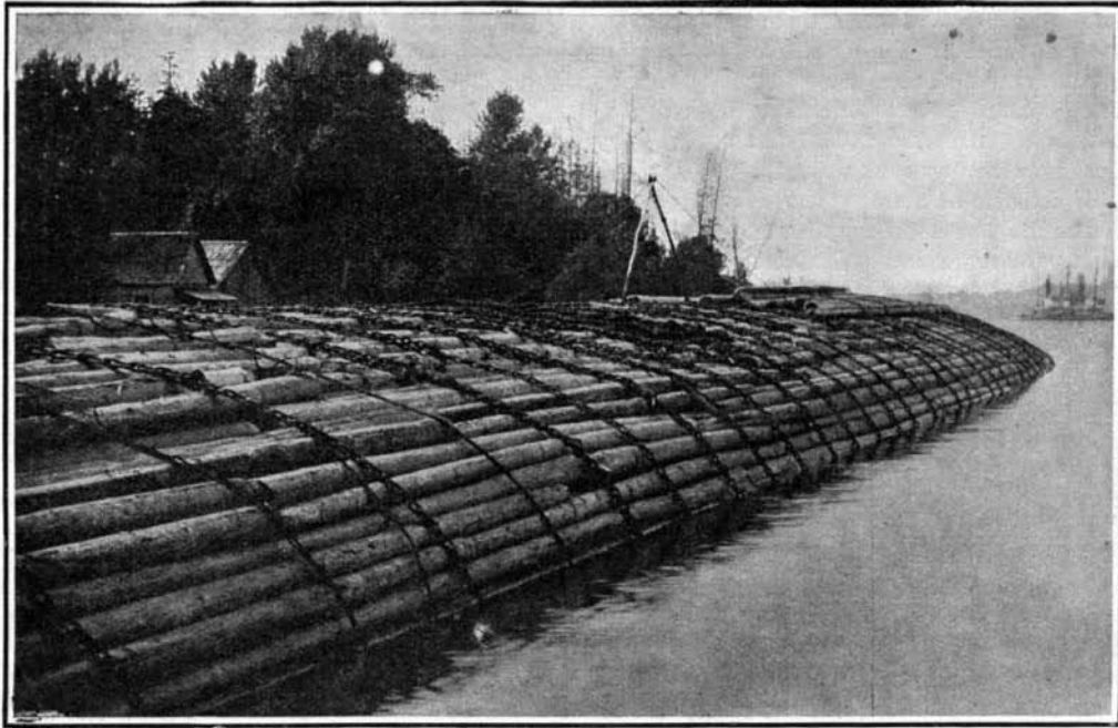
Part of a Completed Raft, Showing the Method of Binding It Together with Chains and Wire Cables.
