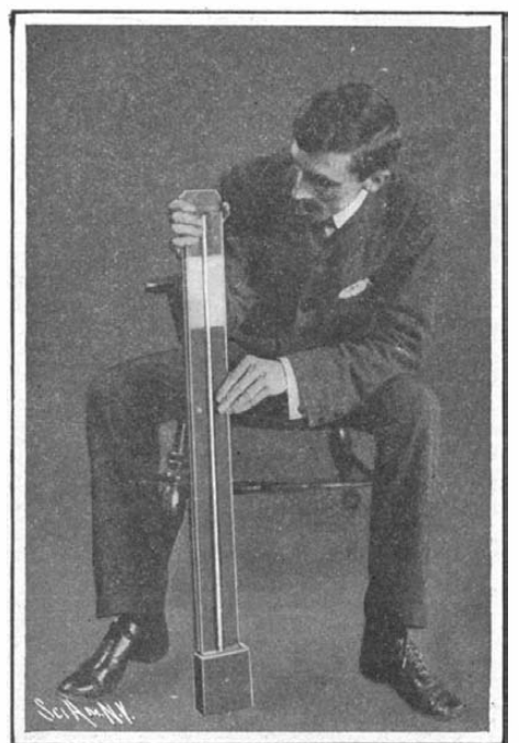
Fastening the Tube to the Frame.
