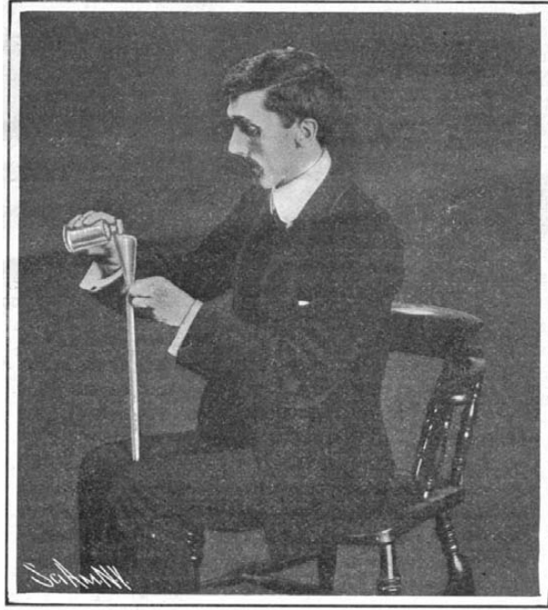
Filling the Mercury Tube.
