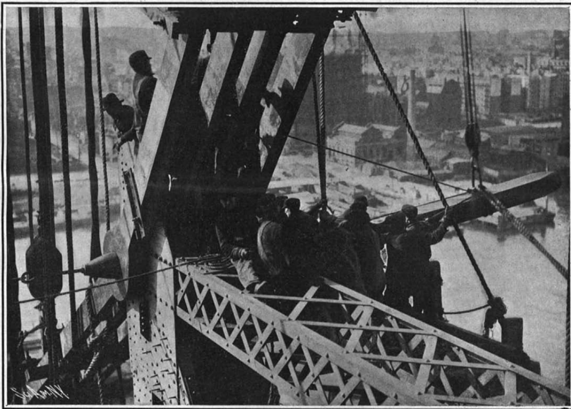
Driving Home a 14-Inch by 5-Foot Steel Pin at Intersection.
