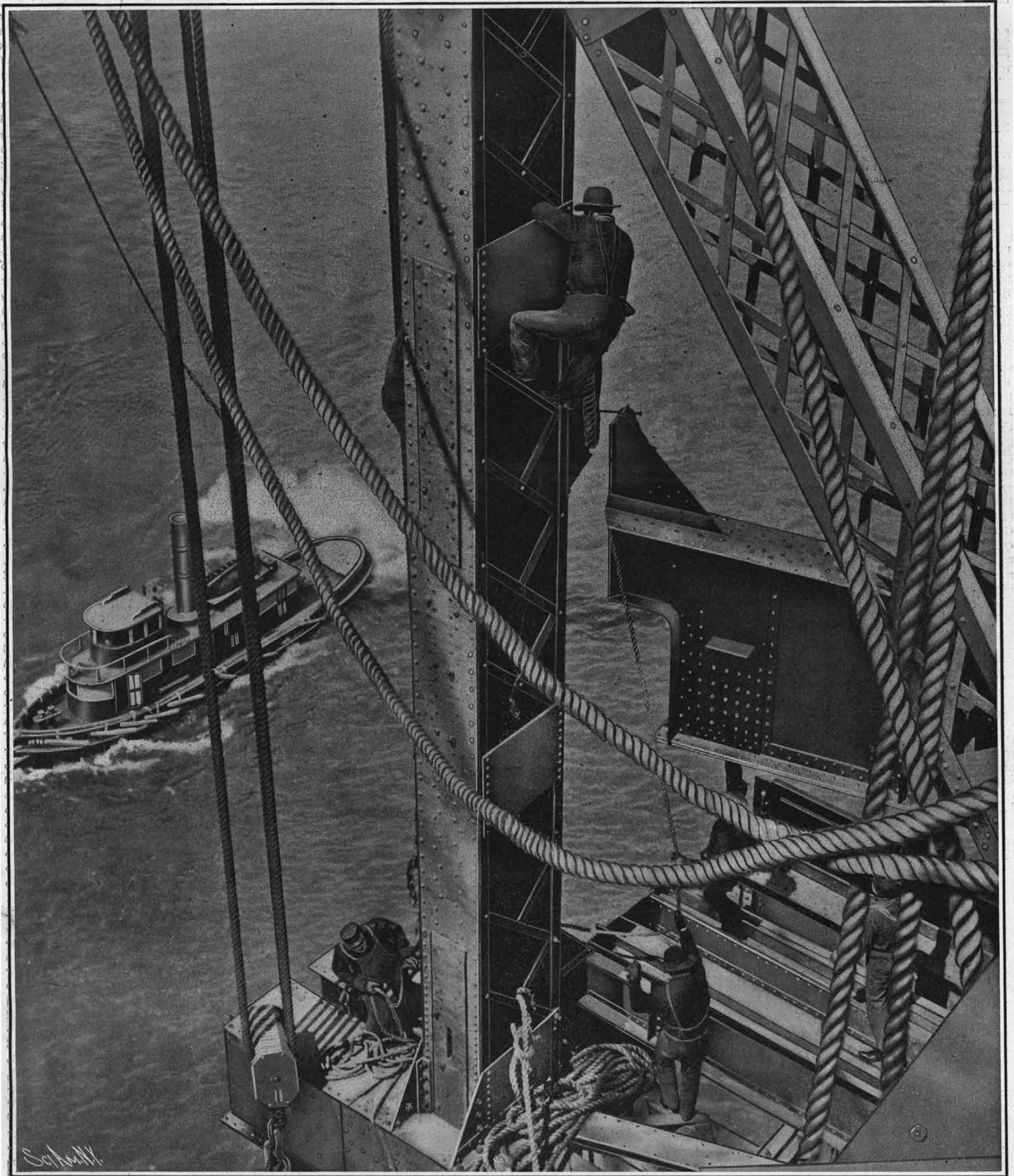
At Work Erecting the Cantilever. The View is Taken 160 Feet in Mid-Air and 500 Feet Out from the Point of Support.
