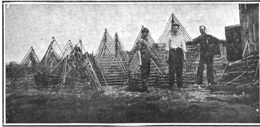
Tetrahedral Units from Which Tower Was Built.
