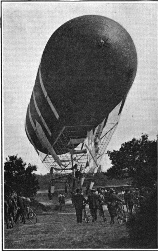
END VIEW OF THE AIRSHIP, SHOWING THE PROPELLERS, RUDDER AND VANES.
