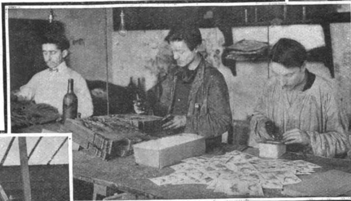
Fig. 4.—Decoration of Cards with the Air Brush.
