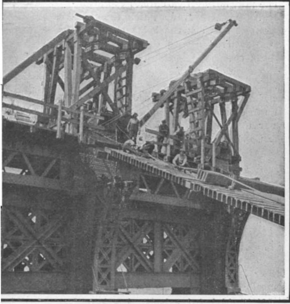
Top of Manhattan Tower, Showing Footway and Temporary Timber Erection Towers.
