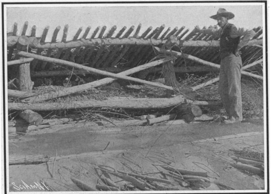
Detail of Abatis. Note the Mats on Which It is Constructed and How Framework is Fastened Together.
