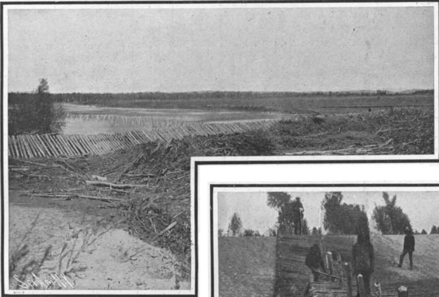
Reversed Abatis. Note Accumulation of Driftwood.
