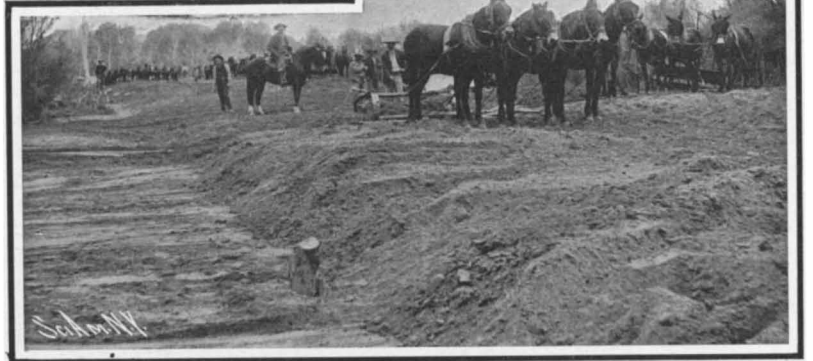
Teams at Work on the Yuma Levee.
