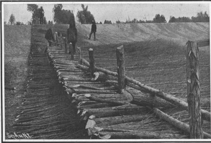
Construction of Brush Fencing and Matting.
