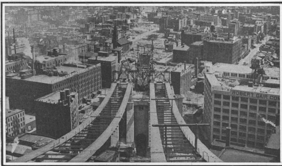
View from Top of Brooklyn Tower. Note the Removal of the Houses on the Line of the Approach.
