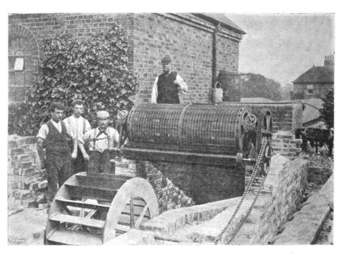
Fig. 17.—Rotary Screen for Crude Sewage at Southall Sewage Works, Isleworth.
