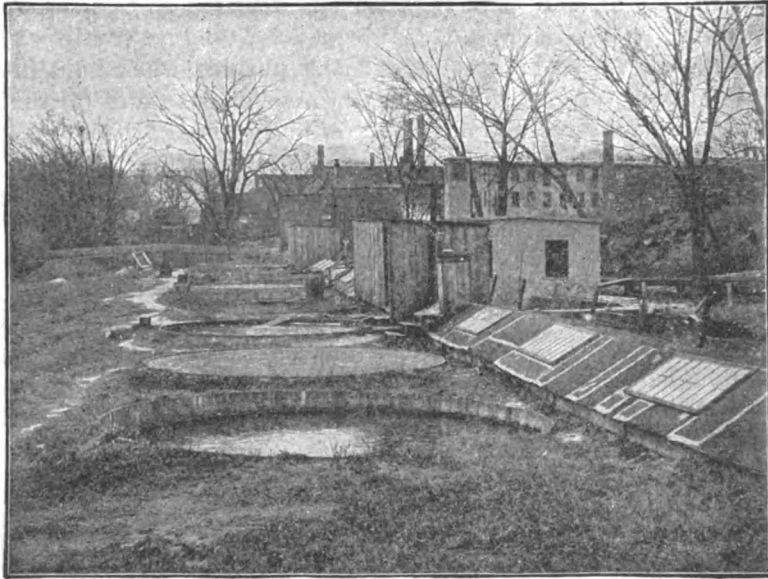
FIG. 22.--VIEW OF LARGE TANKS AT THE LAWRENCE EXPERIMENT STATION.
