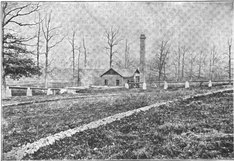
FIG. 109.—GENERAL VIEW OF WORKS FROM SOUTH SIDE OF CREEK.
