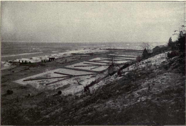
General view Intermittent filtration beds, Lake Forest Plant, \frac{3}{4} of an acre. Rate of flow, 300,000 gallons per acre per day, and upward.
