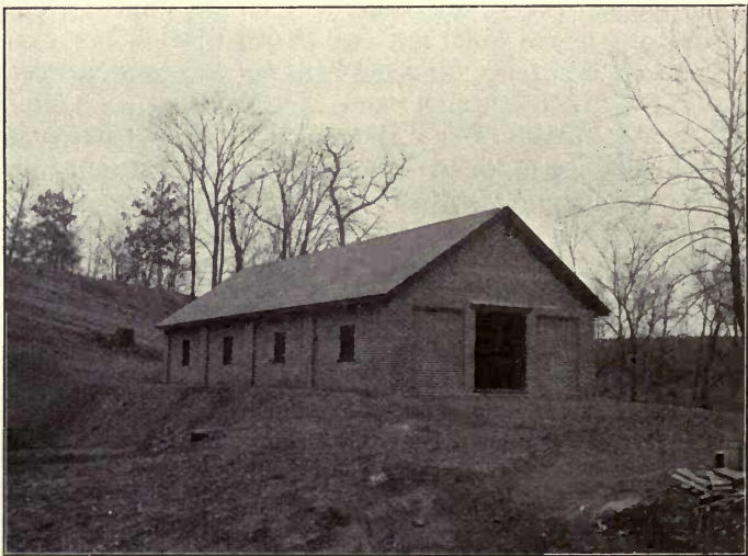
General view Septic Tank at Princefon, Ill. Controlled by 5-compartment system. Liquid capacity, 60,000 gallons. Cost, $3,500.
