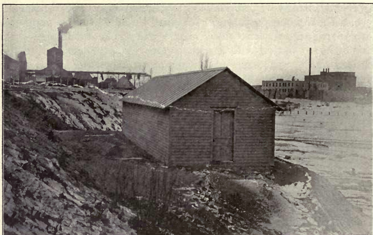
Septic Tank at Holland, Michigan, discharging effluent directly into Black Lake; built entirely of wood. Liquid Capacity, 60,000 gallons. Cost, $1,200. Completed in 1900. First tank using compartment system of control.
