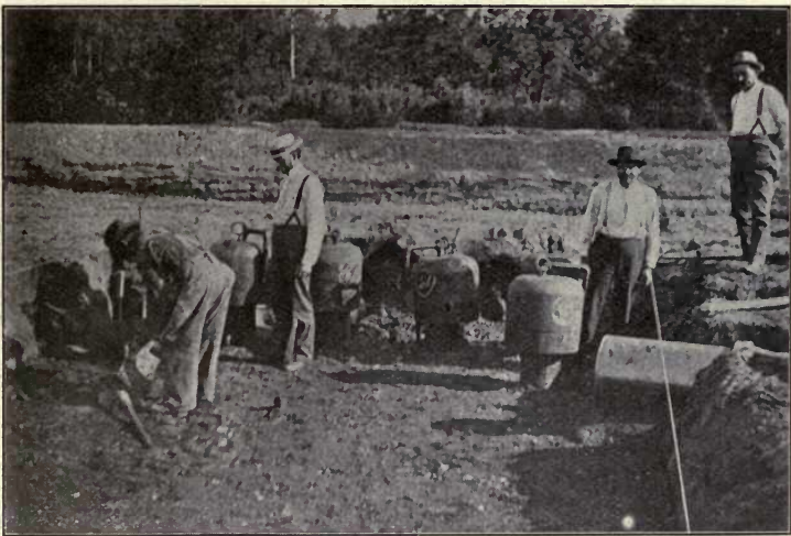
Construction of Automatic Diversion Chamber at Wauwatosa, Wis.
