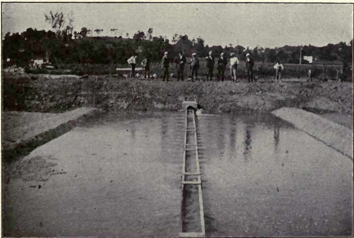
Distribution of Septic Tank effluent upon intermittent filtration beds, at Wauwatosa, Wis. View taken 4 minutes after discharge in diversion chamber. Dose, 6,000 gallons.
