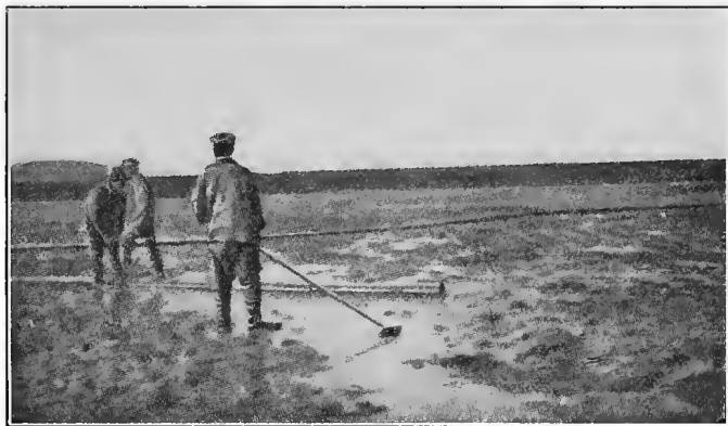
FIG. 29.—Sludge distribution pipes. (Mannheim.)
