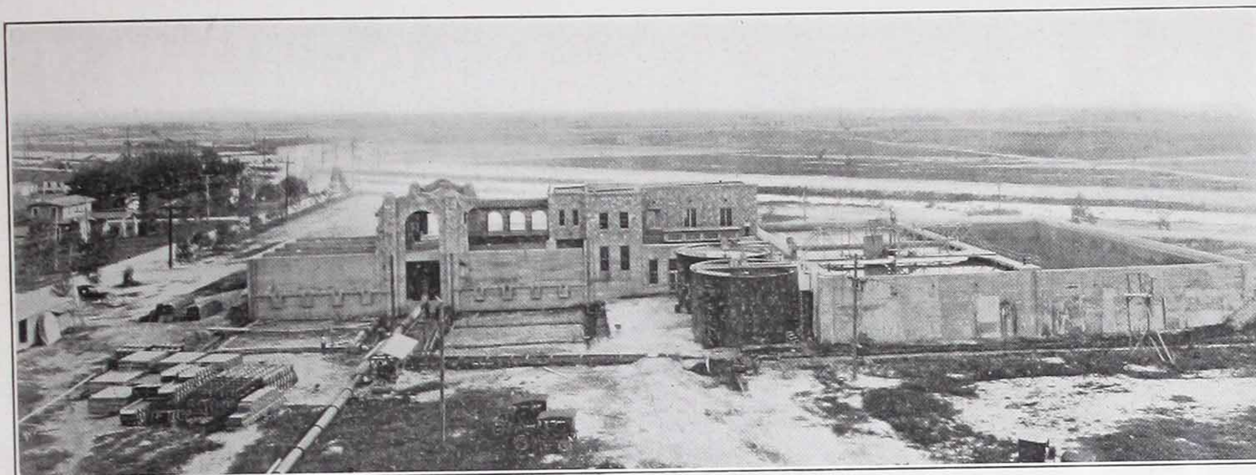
WATER SOFTENING PLANT AT MIAMI, FLA.
