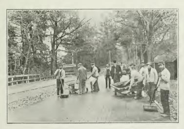
TEST BRICK ROAD AT ITHACA, N. Y. Applying Cement Filler.
