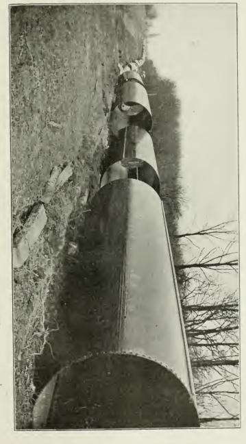
From Valley Stream, Long Island, to Amityville, Long Island (City of New York.) Protected with Sarco Mineral Rubber Pipe Coating. SEVENTY-TWO-INCH STEEL PIPE OF BROOKLYN WATER WORKS.
