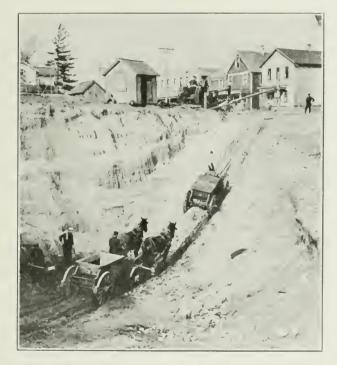
HAULING STUDEBAKER DUMP WAGONS OUT OF GRAVEL PIT WITH TRACTION ENGINE.
