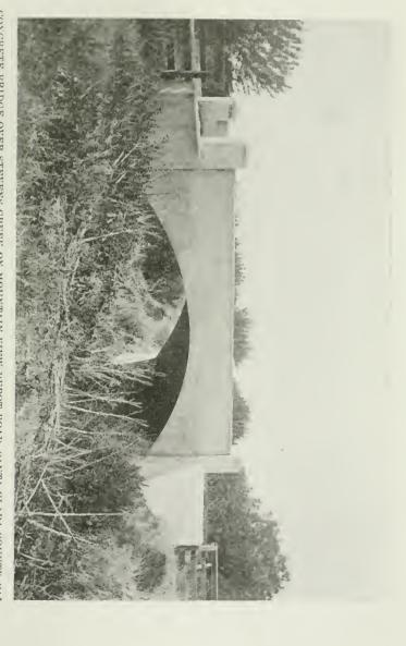
CONCRETE BRIDGE OVER STEVENS CREEK ON MOUNTAIN VIEW DEPOT ROAD, SANTA CLARA COUNTY, CAL. Cost, \$1,473. Span, 36 feet. Roadway, 20 feet. J. G. McMillan, Engineer.
