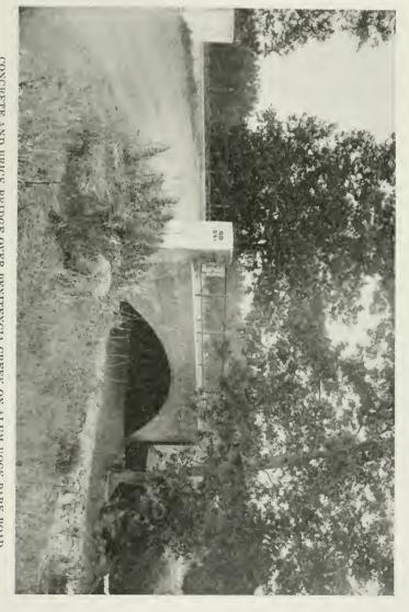
CONCRETE AND BRICK BRIDGE OVER PENITENCIA CREEK ON ALUM ROCK PARK ROAD. First concrete bridge built in Santa Clara County, Cal. Built October, 1891. Cost, \$1,000. Span, 38 feet. Roadway, 28 feet. J. G. McMillan, Engineer.
