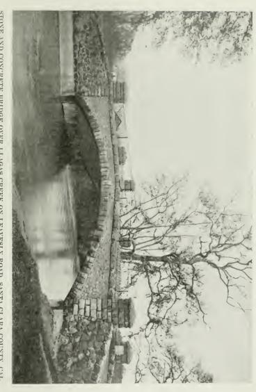
STONE AND CONCRETE BRIDGE OVER LLAGAS CREEK ON LEAVESLY ROAD, SANTA CLARA COUNTY, CAL. Cost, \$3,703. Span, 48 feet. J. G. McMillan, Engineer.
