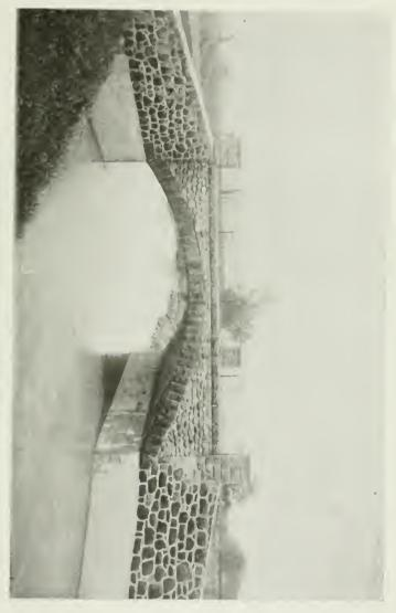
BRIDGE OVER LLAGAS AT OLD GILROY, Span 32 feet. Roadway 20 feet. Cost \$2,950. Built 1902.
