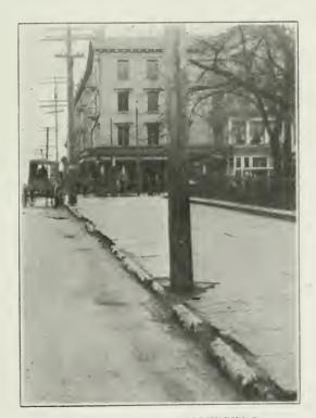
LIMESTONE CURB IN COLUMBUS, O. Almost Disintegrated on E. State St. After 12 to 15 Years Use.
