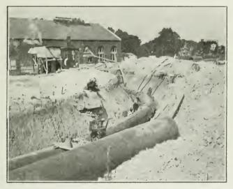
III. TOLEDO FILTRATION PLANT. Riveted Steel Supply Main. Power House in Background.
