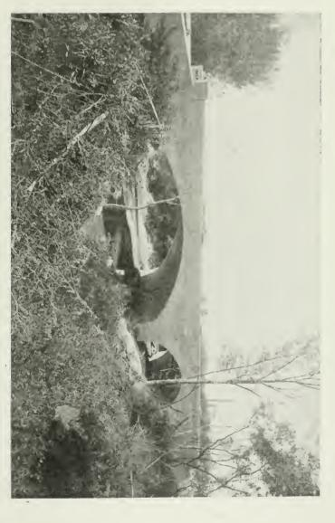
CONCRETE BRIDGE OVER COYOTE CREEK ON BERRYESSA ROAD, SANTA CLARA COUNTY, CAL. Cost, \$13,332. Spans, two-one 68 feet, one 40 feet. Roadway, 68 feet. J. G. McMillan, Engineer.
