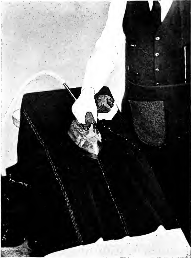
Diagram 3—Pressing Seams. This cut illustrates the correct method of pressing seams as described in Section VI.
