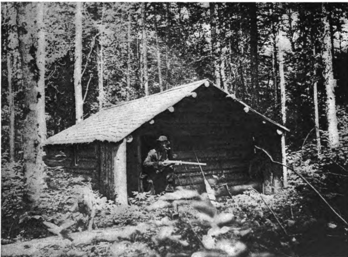
Mouse Tower. The Usual Type of Hunter's Cabin Does Not Always Make Provision for the Storage of Dry Firewood, which was the Chief Design of this Four Foot Projection.
