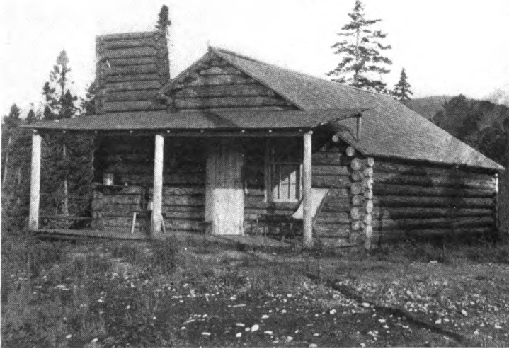
In this Cabin at Beaver Pond, Maine, is Incorporated a Chimney Built of Logs and Lined with Mortar.
