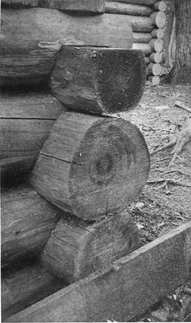
An Expert at Log Cabin Building Can Make a Joint of the Logs that is Almost Perfect.
