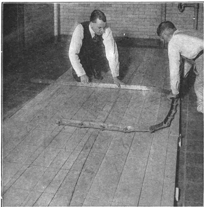
Figure 18.—Picking Up Lines from Mould Loft Floor with a Flexible Steel Template.
