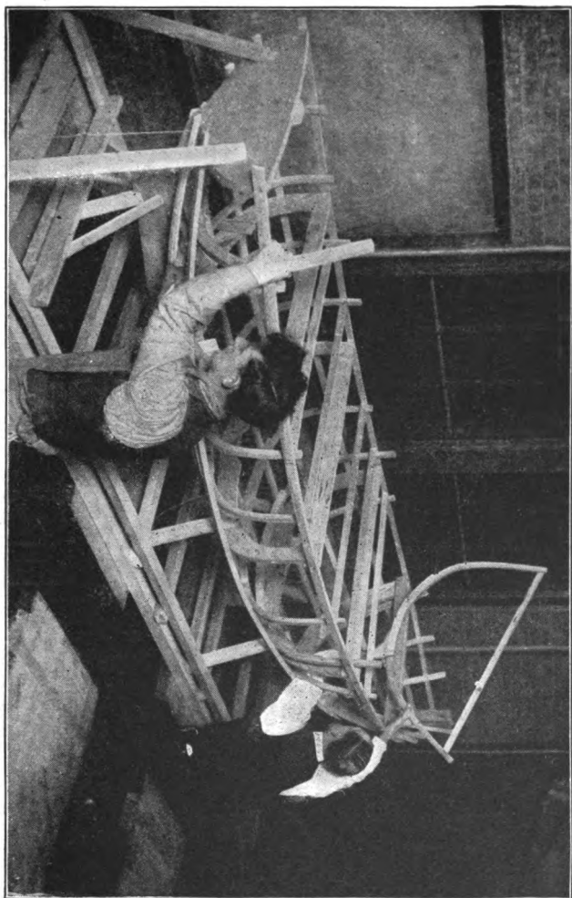
Figure 28.—Fitting Futtocks to Ribbands and Installing Frames.
