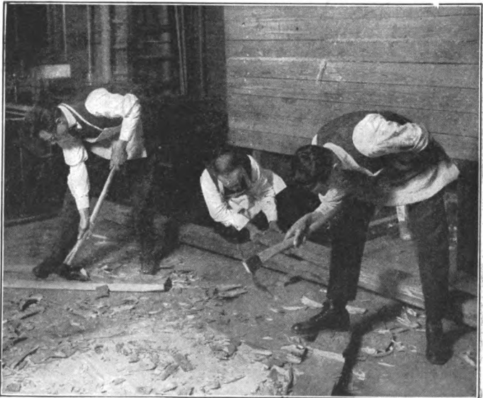
Figure 119.—Scarfig Timber with an Adze.
