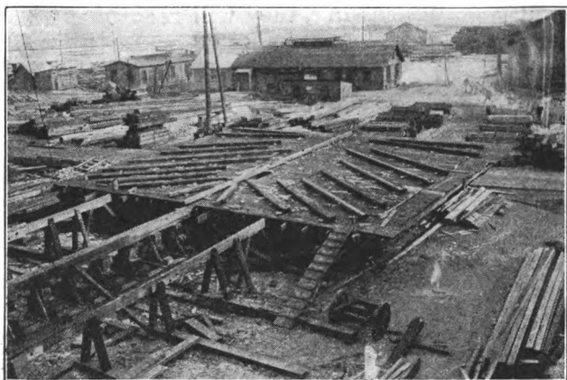
Figure 88.—Assembling Platform, Showing Diagonals.
