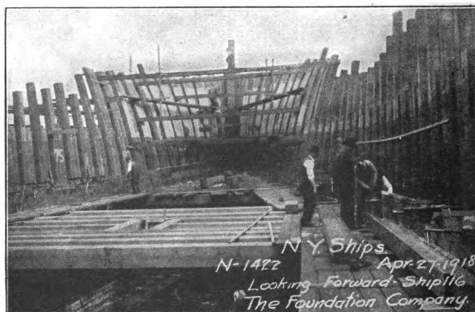
Figure 96.—Looking Forward—Heads of Timbers.
