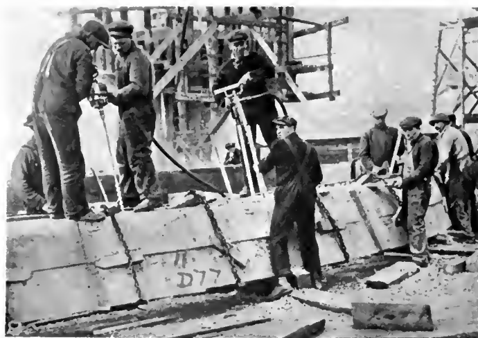
Fig. 74. Assembling a Frame
