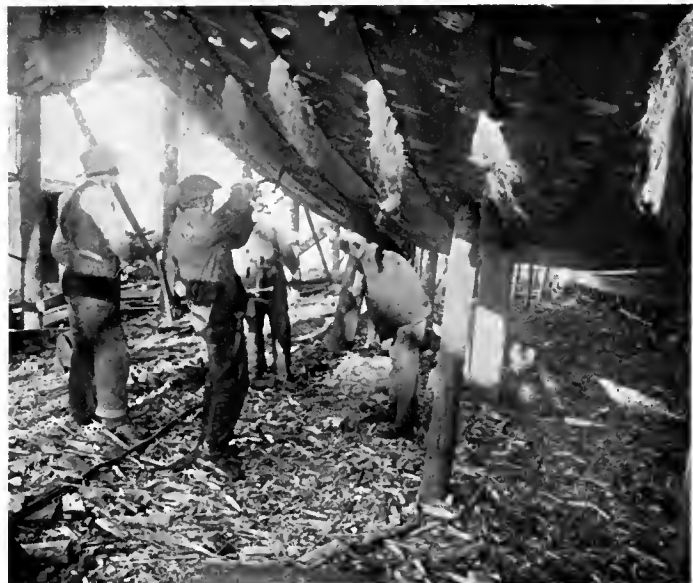
Fig. 93. Caulking Bottom Planking
