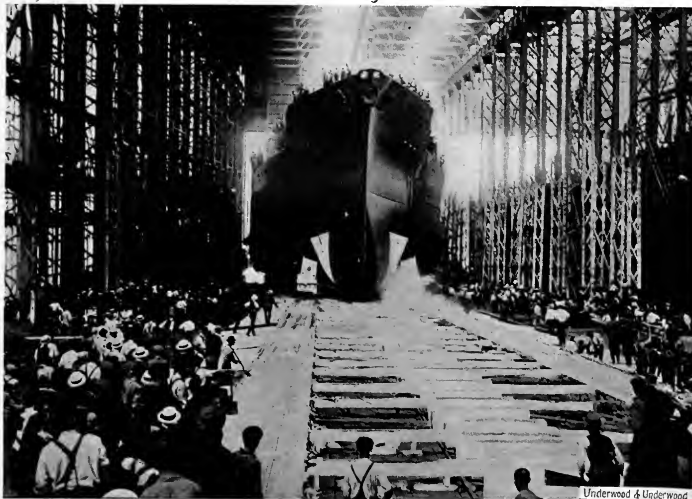
Fig. 57. Steel and Concrete Building Slips, N. Y. Shipbuilding Company, Camden, N. J
