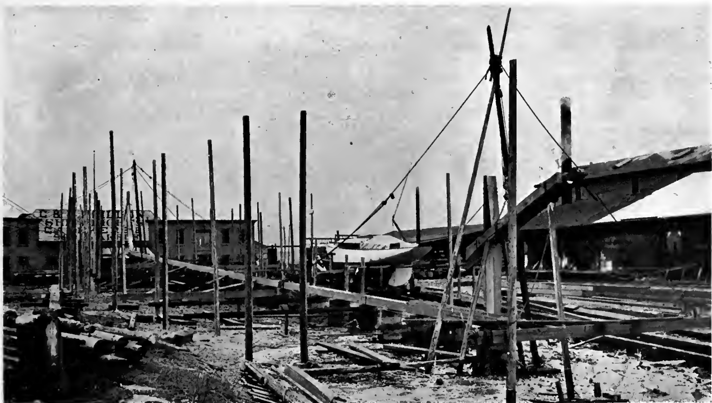
Fig. 82. Setting Up the Stern
