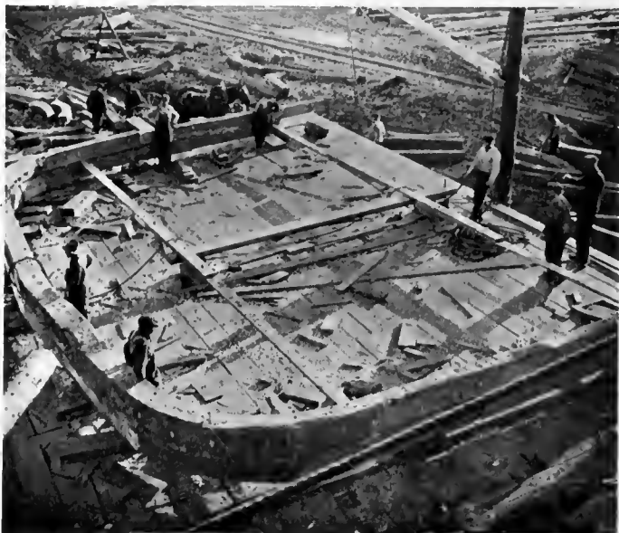
Fig. 75. Assembling a Midship Frame
