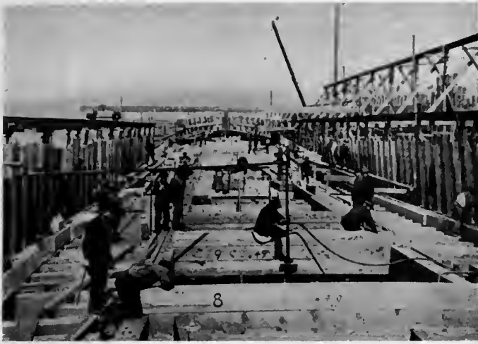
Fig. 53. Deck Framing and Waterways
