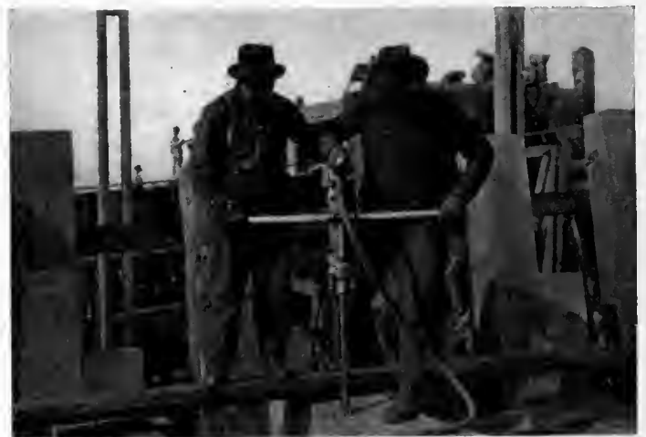
Fig. 81a. The Pneumatic Drift Bolt Driver Hammering Home a Long 1¼-In. Bolt Through a Deck Beam and Its Supporting Sturdy Sill. The Bolt Disappears Into Its Hole With Astonishing Rapidity
