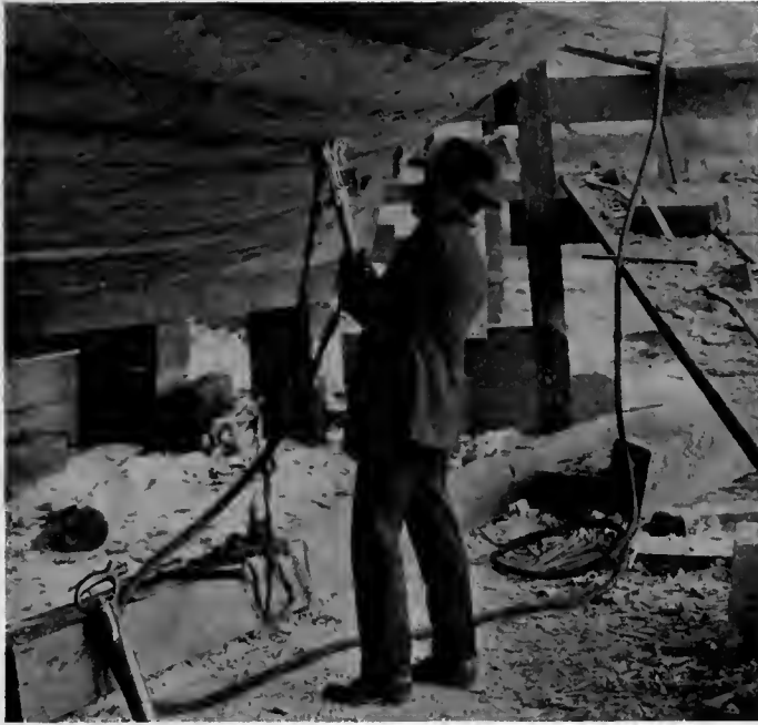
Fig. 99. The Caulking Tool Can Be Held in Any Position and Is Able to Deliver 1,500 Taps a Minute. The Oakum Is Fed Mechanically, so That The Work of "Horsing It In" Can Be Done Rapidly and Thoroughly, No Matter Where the Seam Is Located
