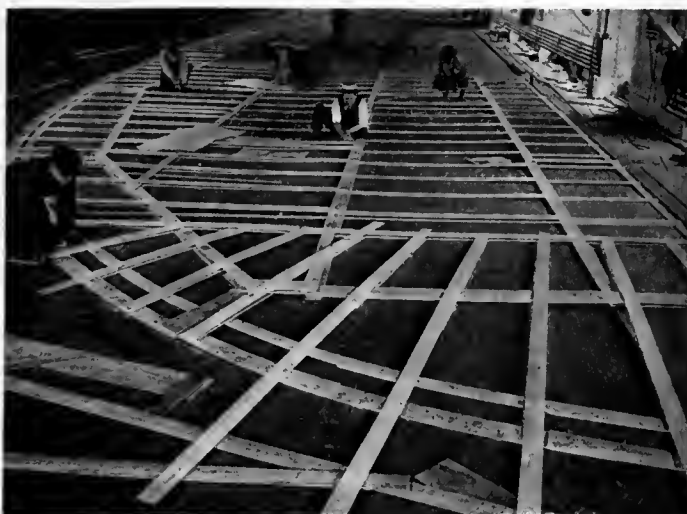
Fig. 73. Mould Loft Work
