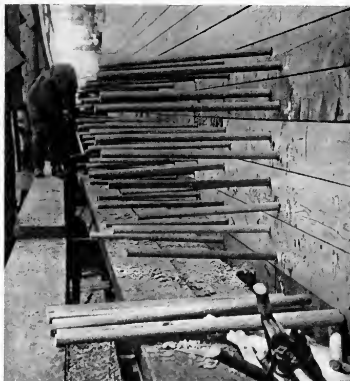
Fig. 47. Treenails Ready to Drive Into Ceiling Frame and Planking
