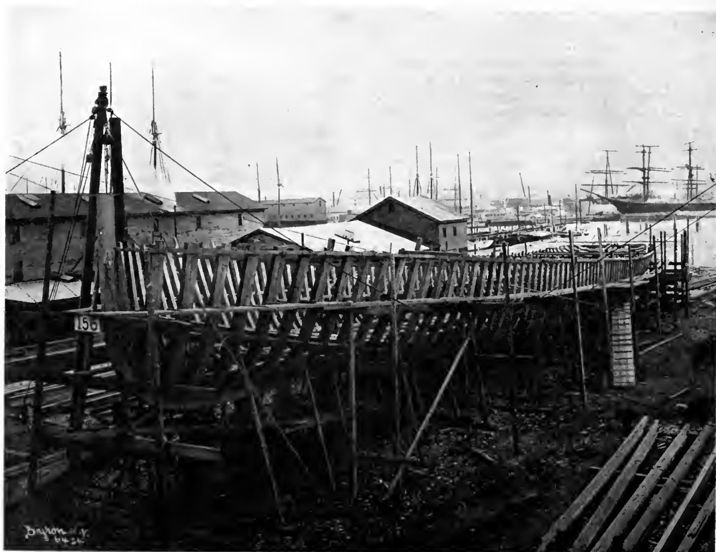
Fig. 90. Framed Ready For Sheer
