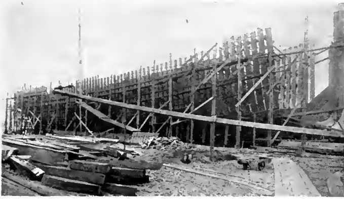
Fig. 79. Stem, Deadwood and Frame Set Up
