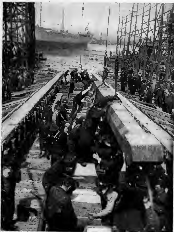
Fig. 29. Laying the Keel of Another Ship as Soon as the Accoms Left the Ways at the Foundation Company's Yard
