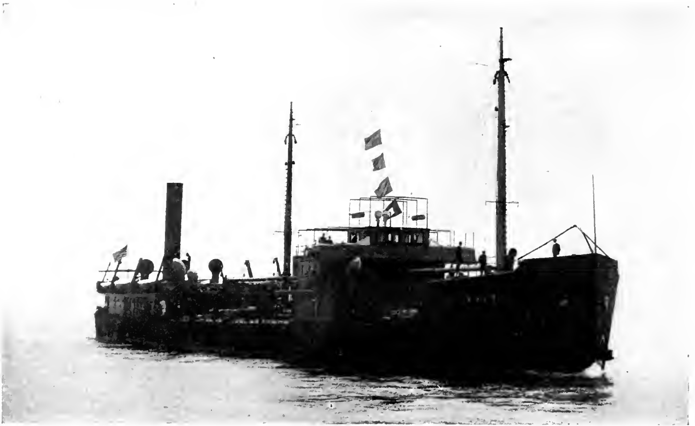
Fig. 149. Faith, the First Concrete-Built Ocean Steamer, Starting Off From San Francisco for Seattle, Tacoma and Vancouver
