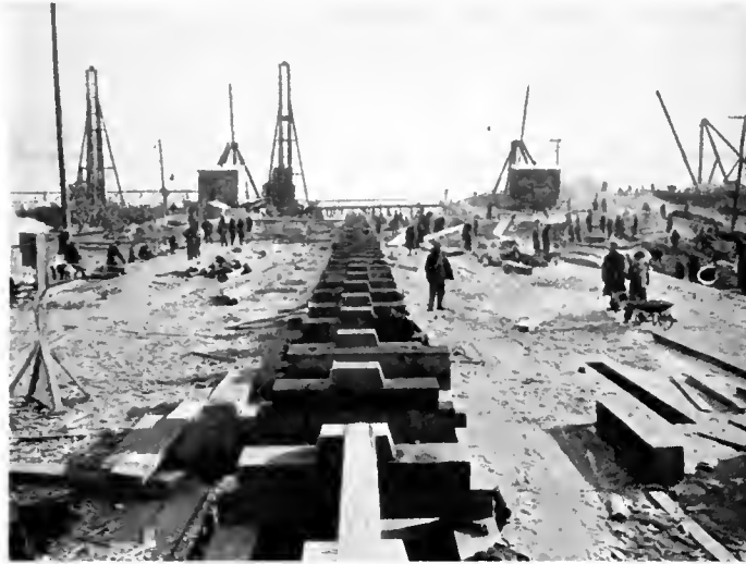
Keel Blocks Being Laid
