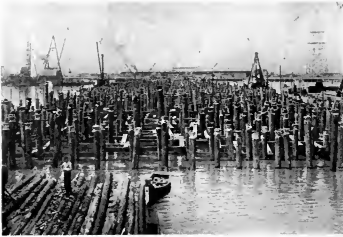
Thousands of Piles Are Driven Into the Marsh on Which to Build the Piers. The Picture on the Left Shows the Piling For Pier and That on the Right Shows Pier Completed and Ready For Use
