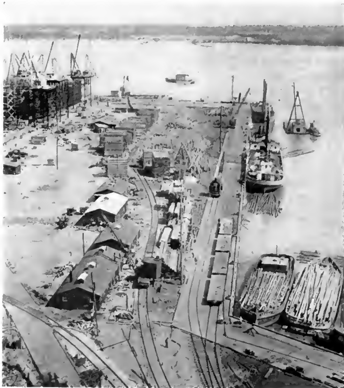
Fig. 72. Traveling Hoists and Tracks in Shipyard
