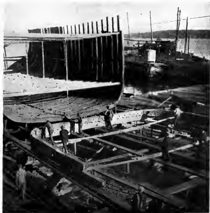
Fig. 76a. Erecting a Midship Frame
