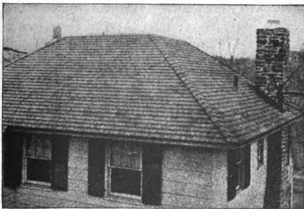
Fig. 132.—Gutter at Rear and Left Side of House
