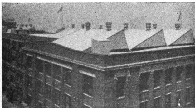
Fig. 96-C.—Saw-tooth Type Roof Skylights Installed for Natural Lighting in Top Floor of Large Building
