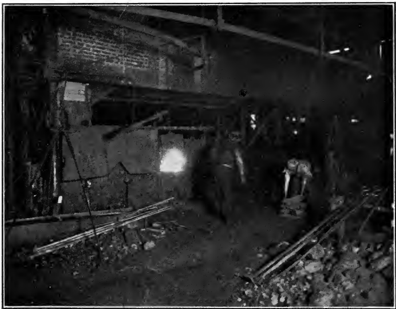
FIG. 44. — CHARGING THE PUDDLING FURNACE.
