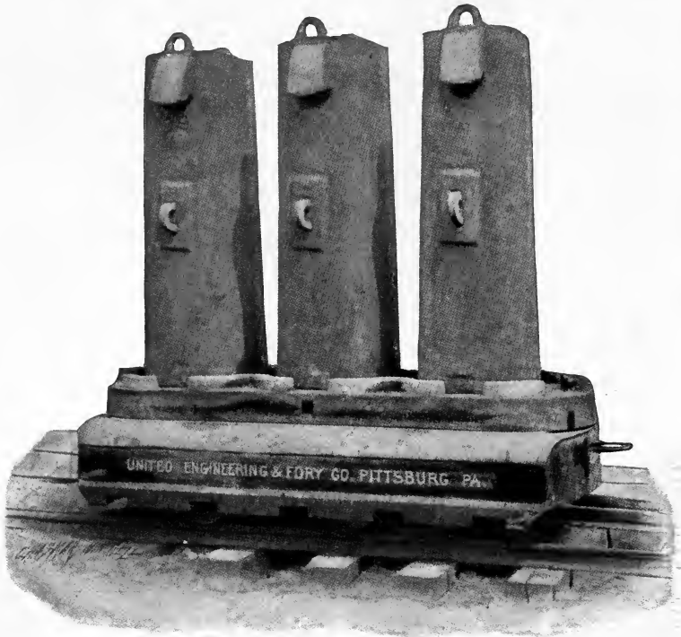
FIG. 78. — INGOT MOLDS, STOOL AND CAR.
