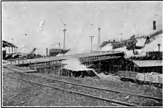
FIG. 24. — UEHLING PIG-CASTING MACHINE.
