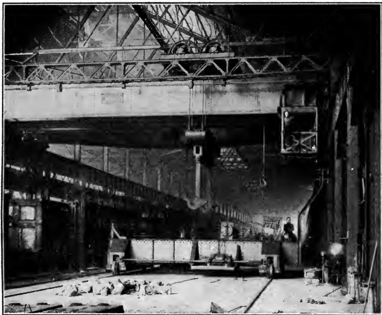
FIG. 92.—OPEN-HEARTH MELTING PLATFORM AND CHARGING MACHINE.
