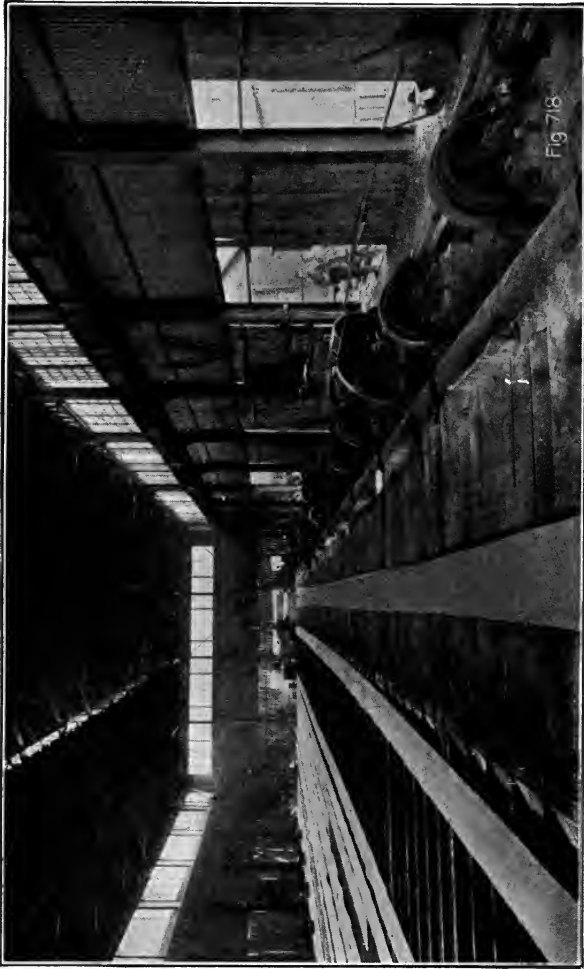
FIG. 167. — SKELP ON A COOLING TABLE.
