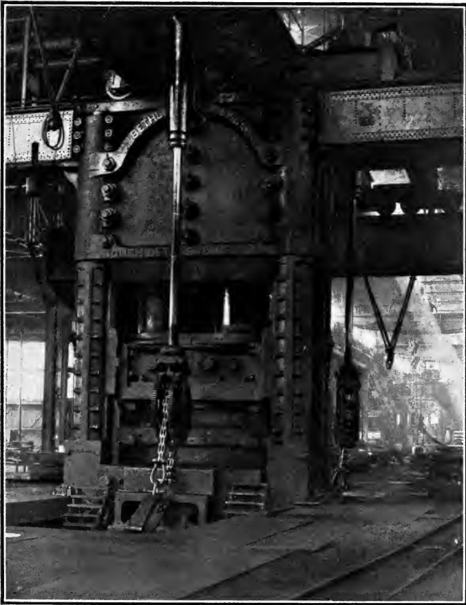
FIG. 177. — FOURTEEN-THOUSAND-TON ARMOR-PLATE PRESS.
