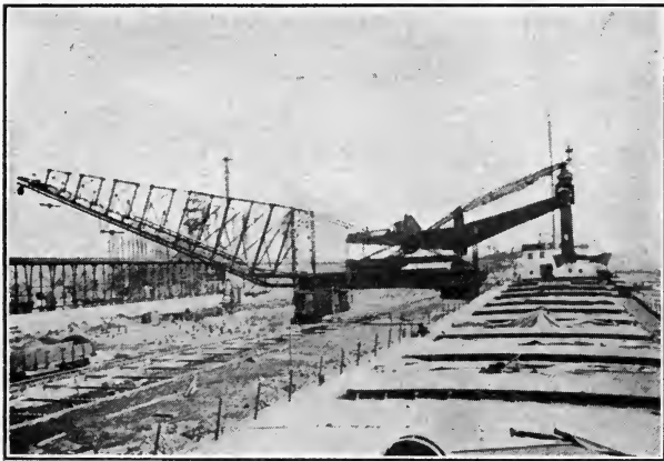
FIG. 13. — HULETT ELECTRIC UNLOADER.
