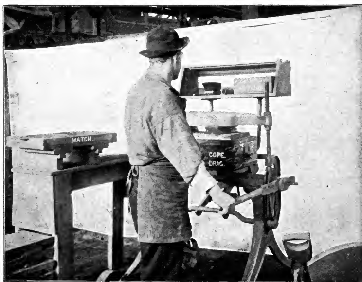
FIG. 205. — POSITION OF MACHINE WHEN PRESSING THE COPE.
