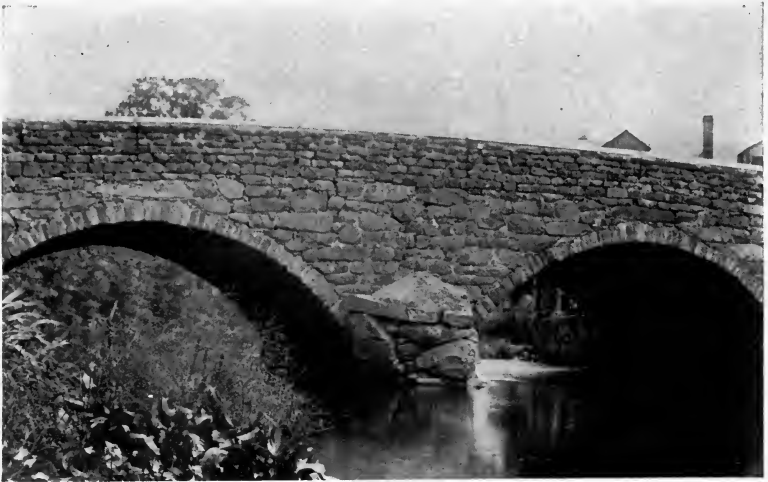
FIG. 30.—Bridge at Ipswich, Mass. Built in 1764. Spandrel Wall Shows Unsquared Stones Laid as Random Coursed Rubble. Parapet Shows Coursed, Quarry-Faced Squared Stones.
