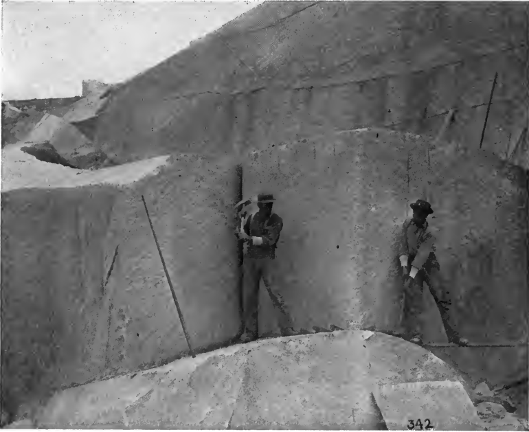
FIG. 1.—“Wood and Water,” or Wedging Up. Note Horizontal Joints.
