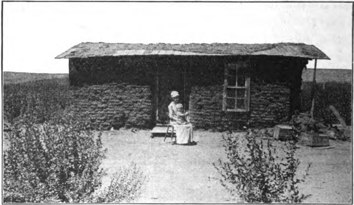
Sod house in Dewey County. This is the sort of home many early settlers in Oklahoma Territory provided for their families. It is as typically an American pioneer home as the log cabin in which Lincoln was born.
