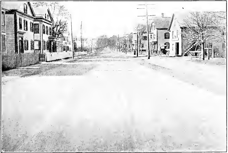
A ROAD BEFORE AND AFTER IMPROVEMENT
