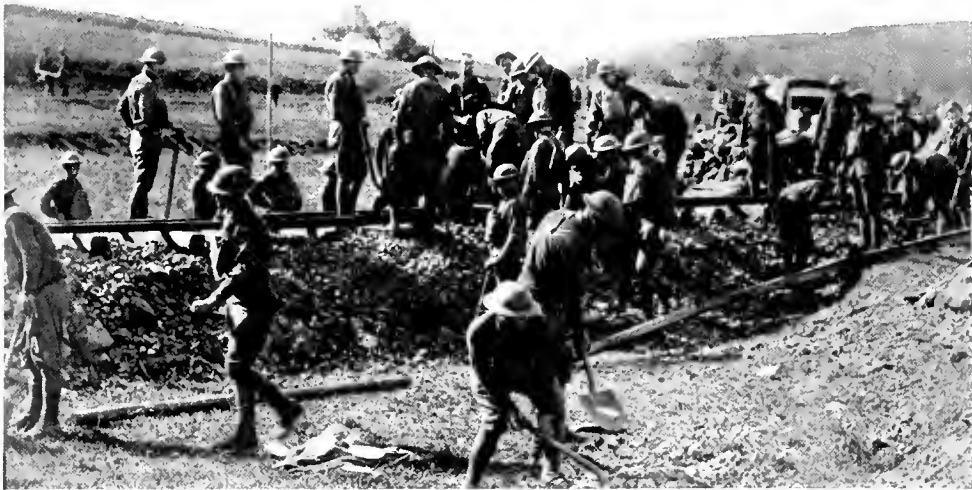
Building Roads in the Recaptured Territory
