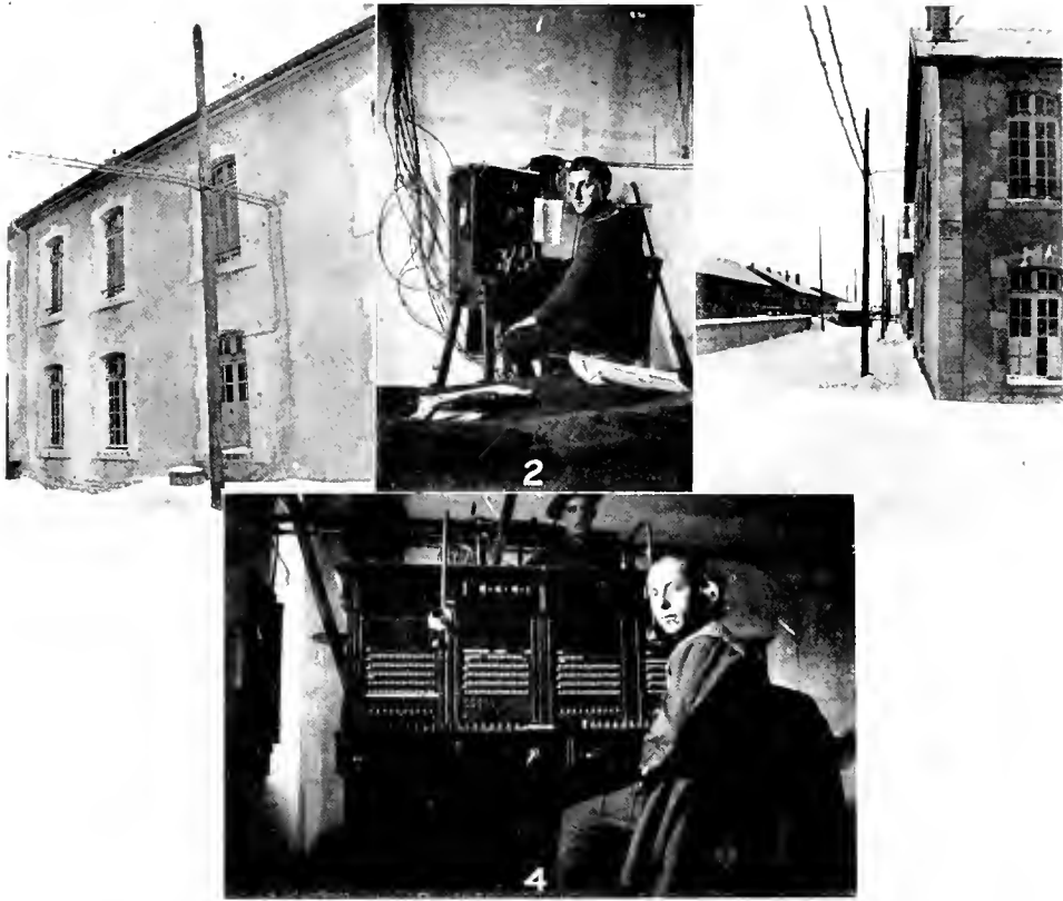
1—Quarters, 2—First Switchboard, 3—Outside Construction, 4—Later Installation.
