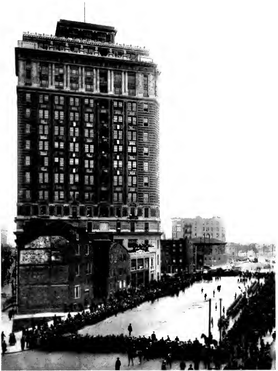
THE REVIEW AT BELL PARKWAY BUILDING
