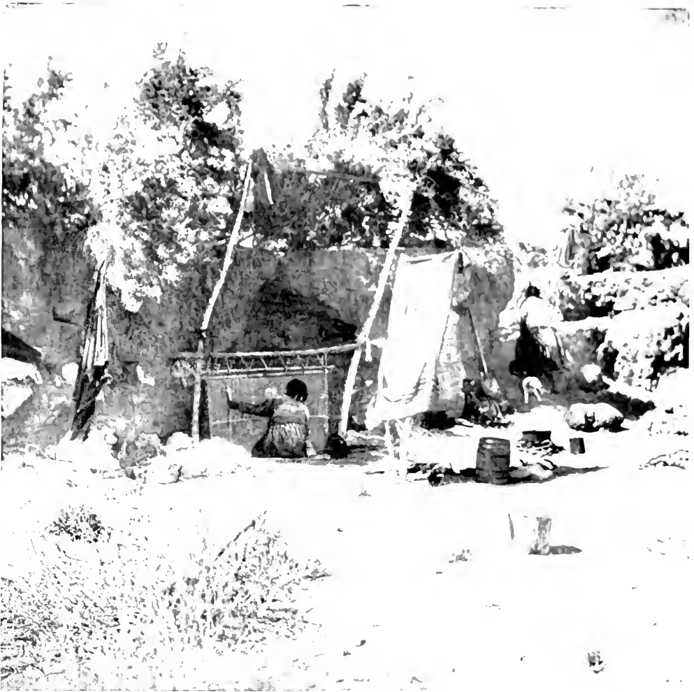
"THE HOGAN, OR HOUSE, GENERALLY CONSISTS OF A FEW TREES DRIVEN INTO THE GROUND TO FORM A SEMI-CIRCLE. THE TOP IS COVERED WITH BRUSH OR A BLANKET, BUT OUTLEN . . . AN ARROYO-BENCH . . . FORMS THE BACK PART OF THE HOUSE."
