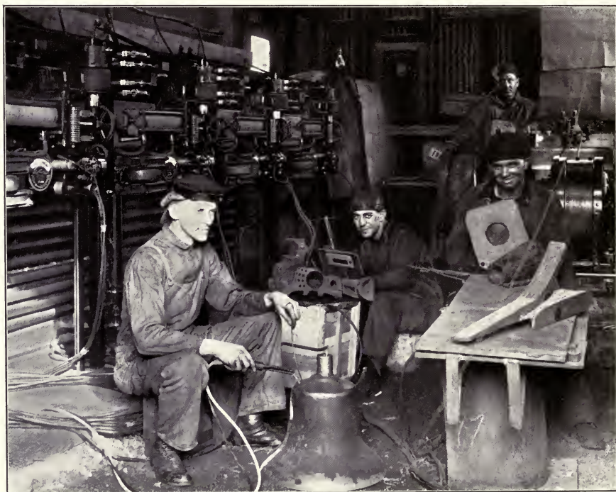
Variety of operations at one and the same time. Four operators welding four different metals, each with a different amperage from a single Generator at the same time and without interfering with each other.
