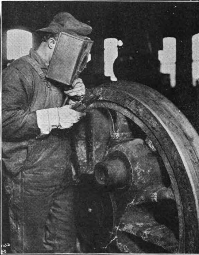
FIG. 121.—Welding Cracked Driving Wheel Spokes.
