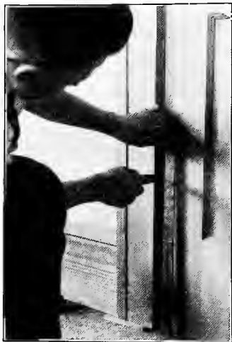
Fig. 135. Locating Hinge Position
