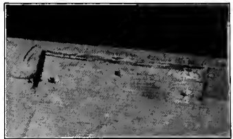
Fig. 139. Gain Ready for Hinge
