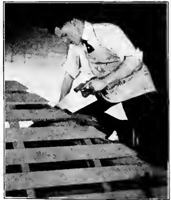
Fig. 92. Sawing Roof Boards
