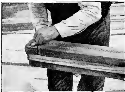
Fig. 31. Marking Joists from Pattern
