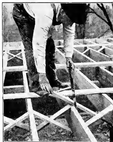
Fig. 23. Cutting Bridging
