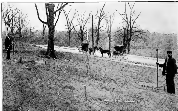
Fig. 5. Taking Sights with Y-Level
