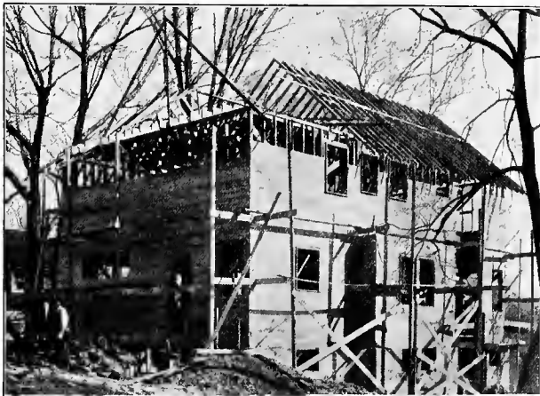
Fig. 42. Raising the Rafters
