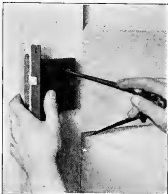
Fig. 142. Locating Knob Spindle Hole
