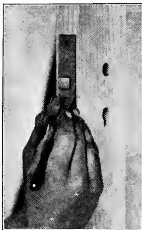
Fig. 143. Locating Selvage Gain
