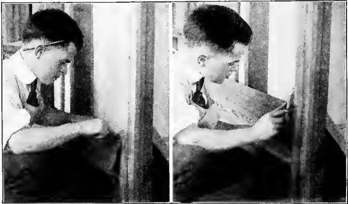
Fig. 114. Marking Length of Siding
