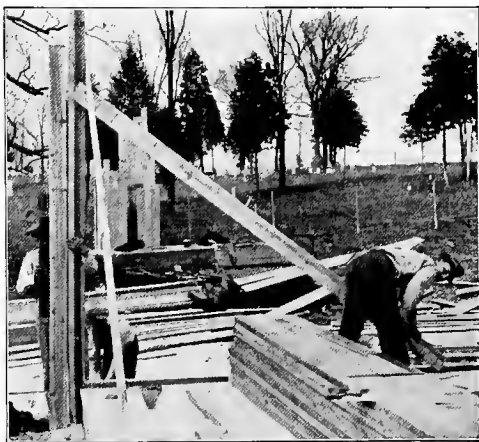
Fig. 33. Corner Post Being Plumbed and Stayed
