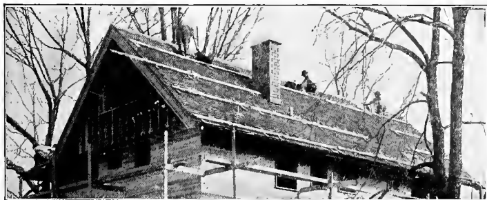
Fig. 104. Shingling. Toe Holds
