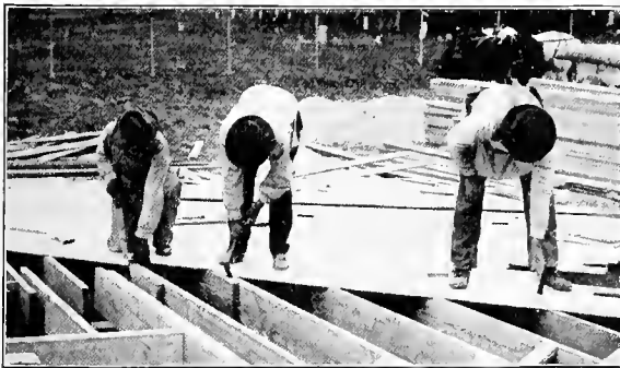
Fig. 27. Floor Frame and Rough Floor
