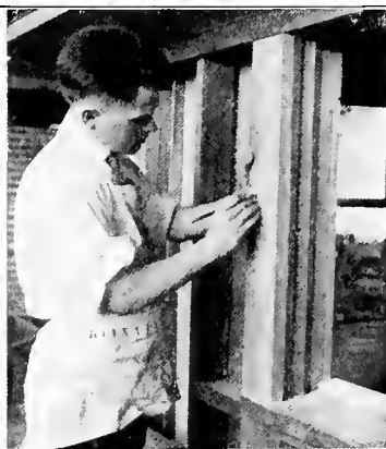
Fig. 113. Using Siding Stick
