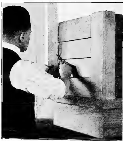
Fig. 117. Scribing against Irregular Surface
