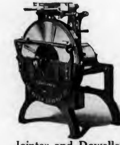
Jointer and Doweller
