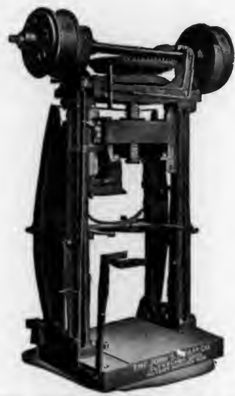
NEW "ECONOMY" (PATENTED) HEADING-UP MACHINE
