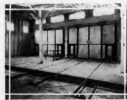
Interior view of Softex kiln.
