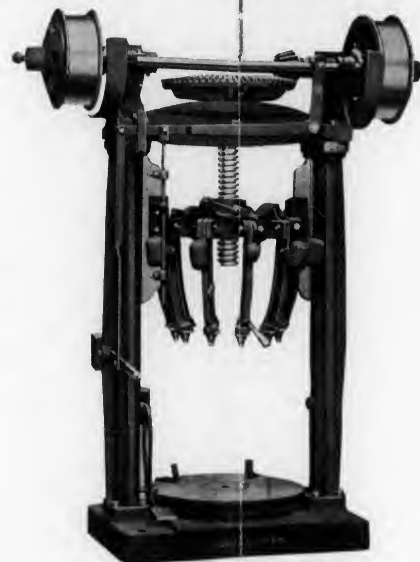
"ORAM" STANDARD HOOP DRIVING MACHINE
