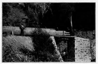
FIG. 29.—Assembling parts of redwood stave pipe.
