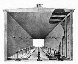
FIG. 69.—Interior of a drying chamber.
