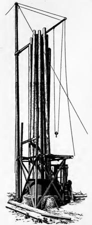
FIG. 76.—Open-tank for Butt treatment of long poles. From "Preservative Treatment of Poles," Kempfer (United States Forest Service, Bulletin No. 84).
