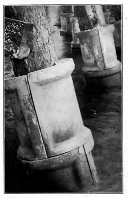
FIG. 61.—Piles protected by pipes and sand.<sup>2</sup>
