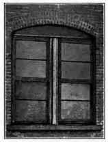
FIG. 48.—Wired glass window in metal sash.<sup>3</sup>
