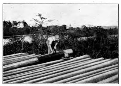
FIG. 75.—Treating poles by brush method.<sup>1</sup>
