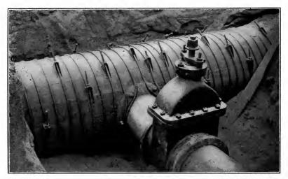
FIG. 30.-Completed redwood stave pipe with gate.
