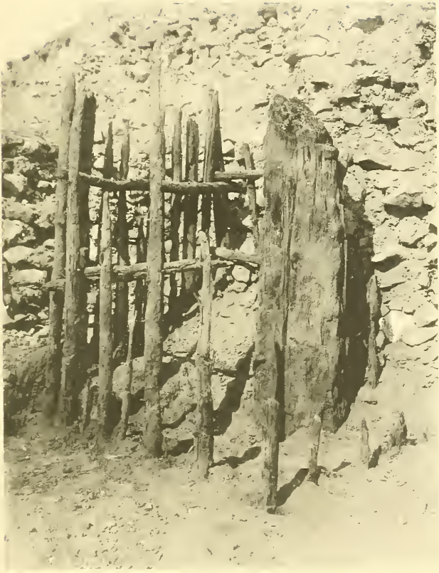
CEDAR BEAMS AND POLES TEMPLE OF QUETZALCOATL
