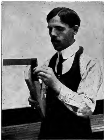
Fig. 102. Testing a Round End.
