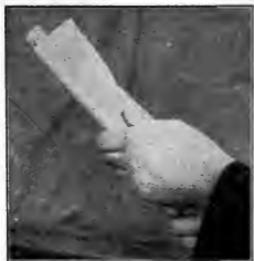
Fig. 126. Sandpapering a Cylinder.
