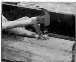
Fig. 28. Using a Nail for a Nailset.
