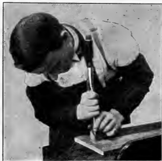
Fig. 43. Chiseling an End.
