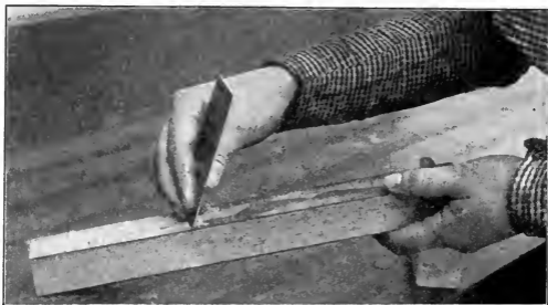
Fig. 49. Scraping Thick Places in the Finish.
