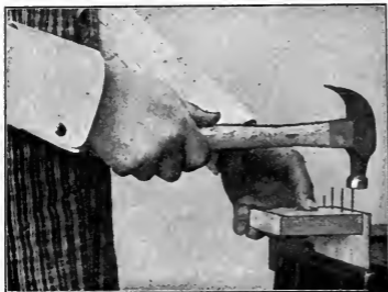
Fig. 108. Nailing a Rabbeted Corner.
