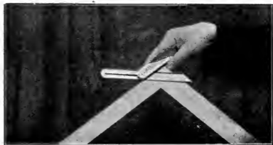
Fig. 204B. Setting a Tee Bevel.
