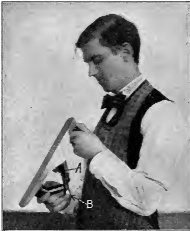
Fig 169. Sighting the Bottom of the Iron Plane.
